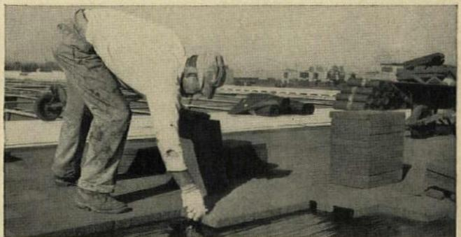
**FOAMGLAS Insulation** clears the air beneath this roof. Cold outside temperatures contrasting with a hot, humid interior atmosphere, had caused a fog-like condensation. FOAMGLAS roof insulation eliminated the problem. And the incombustibility of FOAMGLAS was an important extra-benefit here.
