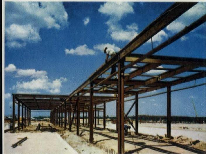
Key factor in concourse design was use of J&L 14-inch Light Beams as purlins. Span between rigid bents varies from 19' 7" to 24' 0". Formed metal decking, which supports insulation and built-up roofing material, is welded to the purlins. Purlins and girders also support a maze of concealed piping.
