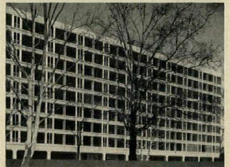
Plaza" ultimately will include four such apartment structures for a total of 512 units, a 17-store shopping center, and a community plaza. The buildings, designed by I. M. Pei & Associates, are of reinforced-concrete construction with windows almost floor to ceiling. An in-swinging, railed window in each room gives the feel of a balcony. At the ground level, each building has a glass-enclosed lobby surrounded by a colonnade. Apart-
