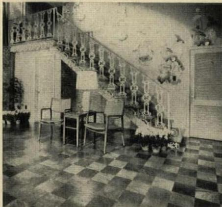
stretching, shrinking, or buckling when laid as a floor. The millions of expansion joints created in the stretching process allow the wood to expand and contract internally, leaving it dimensionally stable. The 1/8"-thick tiles have a six-coat factory pre-finish and can also be used on walls or counter tops. Flexible enough to be
