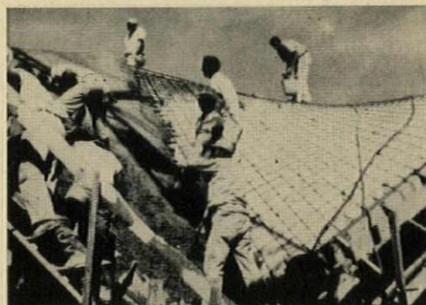
Styrofoam is laid over wood form and covered with reinforcing.
