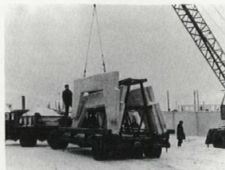
Typical scenes from apartment house construction sites where prefabricated concrete parts are being delivered for erection.
