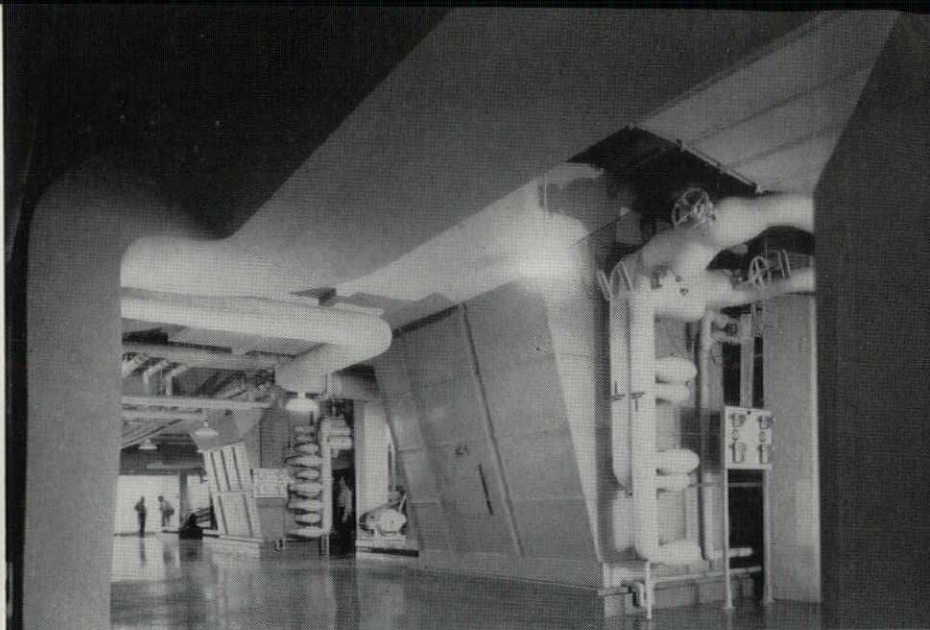
Air-conditioning and ventilating equipment inhales and exhales as much as 200,000 cu. ft. of air per minute.
