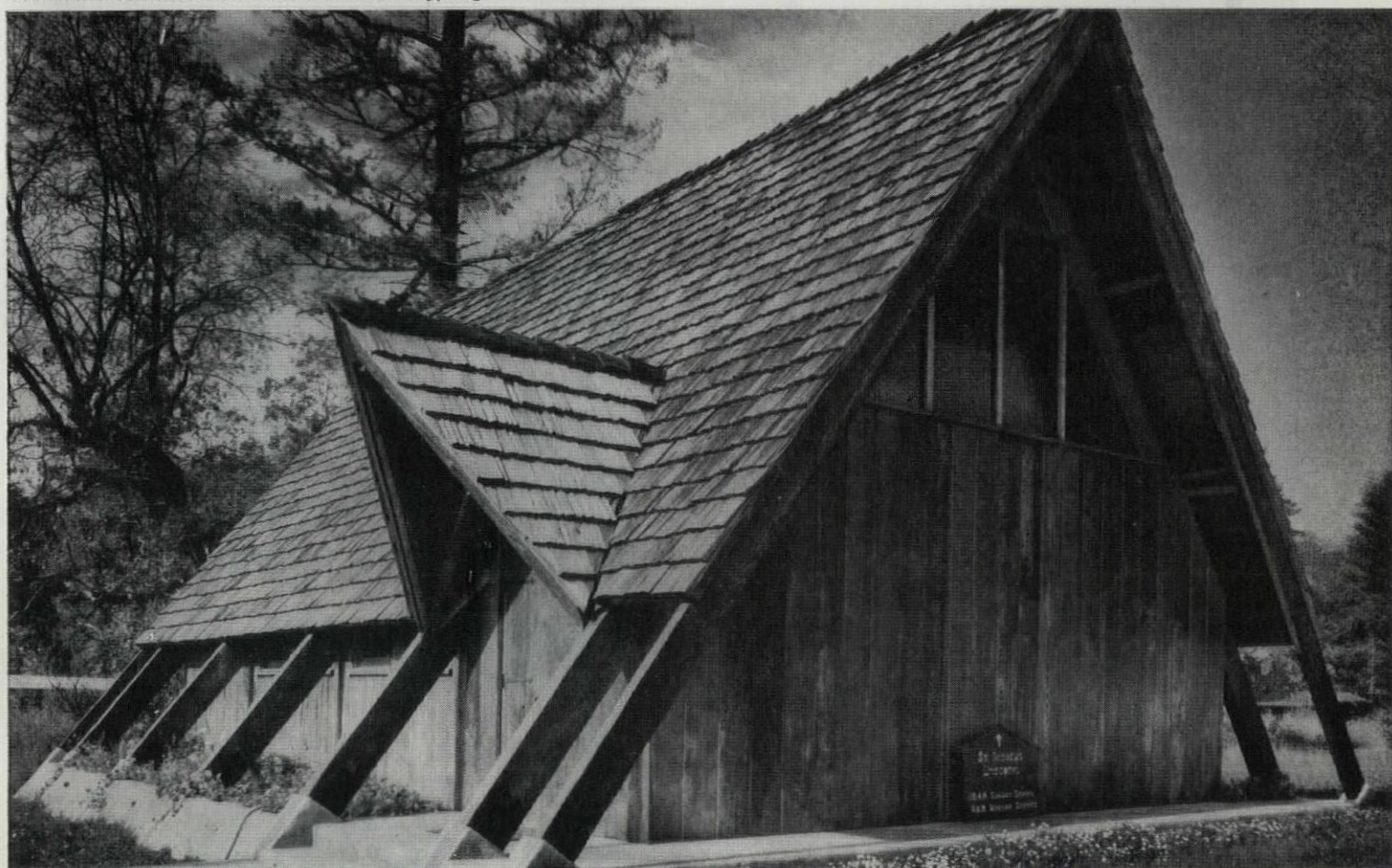
Economy in small church design uses the wood A-frame for maximum space inside. Outside, the naturally weathered shingled roof, heavy A-frame supporting members, and board siding create a welcome site for worship. Gerald Matson, architect.
