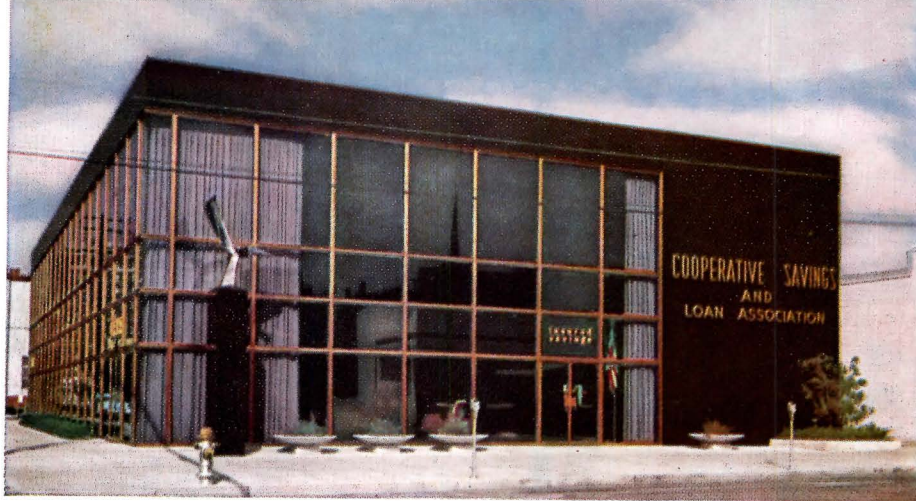
▲ Cooperative Savings & Loan Association , Wilmington, N. C. Architectural Bronze lends to this modern building of glass and metal a feeling of warmth and dignity. Nearly all the architectural metals used on the structure are extruded Bronze, including mullions, glass stops, doors, and air-conditioning grilles. ARCHITECT: Leslie N. Boney, Wilmington, N. C. FABRICATOR: Newman Brothers Inc., Cincinnati.
