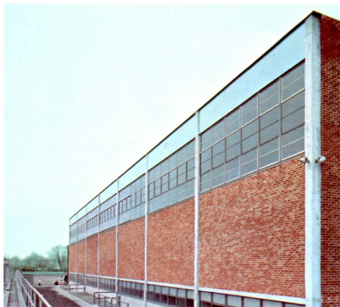
Hammered Coolite Wire Glass spans western elevation in new gymnasium of Belleville Township High School, Belleville, Illinois. Associated Architects: Charles E. King & Wesley W. Chorton.
