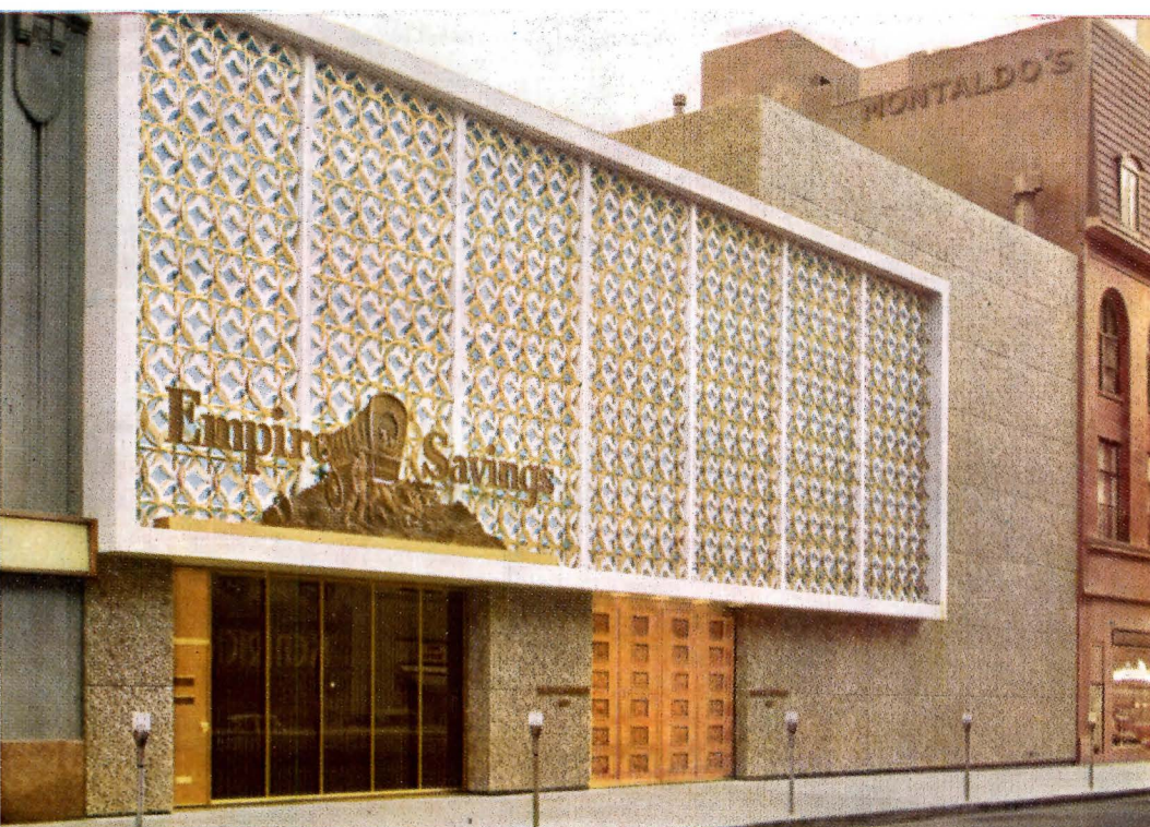
▲ Empire Savings Building & Loan Association , Denver, Colo. The architectural screen dominating this facade consists of 24" dia. circles made from 1" square Red Brass tubes. Where rings intertwine, cast Nickel Silver inserts with sandblasted sides and polished faces accent the design (see drawing above, right). ARCHITECTS: Raymond Harry Ervin & Associates, Denver. FABRICATOR: William G. Zimmerman Architectural Metals, Inc., Denver.
