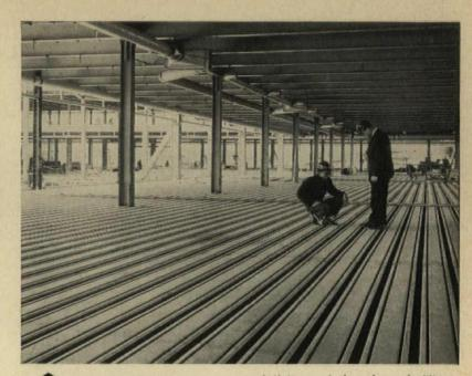
Mahon 3-in. beam depth M-Floors, during erection in eastern Pennsylvania project. General Contractor: McCloskey, Inc., Phila. Artist's rendering of new facility for steel company. M-Floors permit quick...and flexible...electrical wiring of the facility. Architects: McKim, Mead & White, New York
