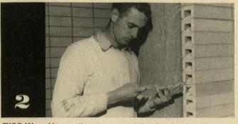
TIES IN ... Many wall sections were left unfinished for other work to progress. For continuous reinforcement, Keywall was used. Bill Revers of Crouch-Walker, shows the Keywall "tails" to be tied in later. Only Keywall can be tied in. Only Keywall is flexible enough to accommodate variations in mortar joint levels.
