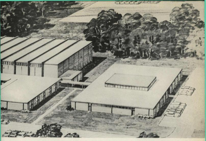
Steel is used extensively throughout the Georgia National Guard Armory, not only as a structural system, but also as frames for windows, canopies, and glass curtain walls. Architects and Engineers: Thomas-Driscoll-Hutton. General Contractor: Hugh Jackson. Steel Fabricator: Owen Steel Company. Steel Erector: Steel Erectors, Inc. The major portion of the 310 tons of structural and miscellaneous steel was supplied by Bethlehem.
