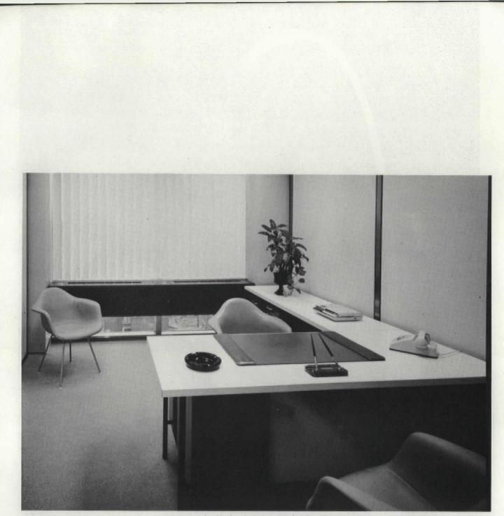
A typical assistant manager's office illustrates the interior treatment of the curtain wall. The air-conditioning enclosure is raised above the floor with a clear-glass panel below it.
