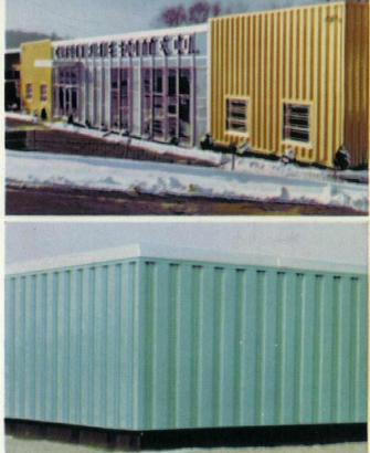
(top) EGSCO insulated wall panels with Colorgard in tan and gold were erected on this recently completed Williamsport, Pa., plant of The M. W. Kellogg Company, where the Power Piping Division is located, including engineering, research and field erection and the manufacture of power piping systems. Engineer and architect is Lester B. Knight and Associates, Inc., Chicago.
