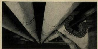
FOAMGLAS Stay-Dry Pipe Insulation provides the important benefits of FOAMGLAS for all building service lines; iced water, chilled water, low-pressure steam or dual temperature runs. In addition to the vapor and moisture protection, the insulation is fireproof, will not slump or sag, and will not compress around saddle supports.
