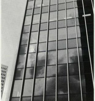
Green-tinted glass windows and spandrels of the 4 Gateway Center Building in Pittsburgh, by Harrison & Abramovitz, are framed by mullions of 16-gage Type 302 stainless steel and horizontal strips of gray stainless steel, colored by a recently developed modified acrylic resin.
