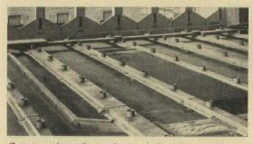
Construction photo shows A-E cells resting on steel pipe supports.
