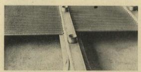
Detail shows corrugated plenum form and round, preset inserts of system.
