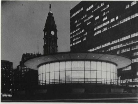
Built for the City of Philadelphia and its Convention and Visitors Bureau, this Hospitality Center by Architects Harbeson, Hough, Livingston & Larson is enclosed by glass walls framed in nickelfinished Type 302 stainless steel. The circular roof is supported on steel arms cantilevered from a concrete stem.
