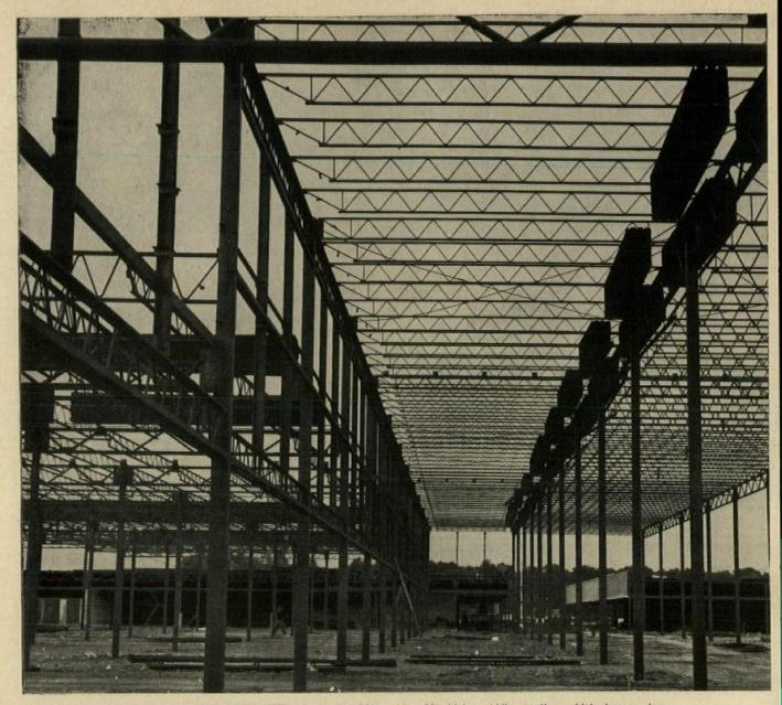
TWO STORIES OF INTERLOCKED STEEL frame the 320' wide, 25' high, middle section which houses two department stores. Standardized, interlocking girders and purlins required no bolting, riveting or field welding — reduced engineering, fabrication and construction costs — advanced completion and occupancy dates.
