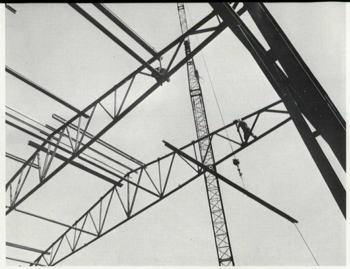
Erecting a pre-engineered truss frame with a 90-ft span.
