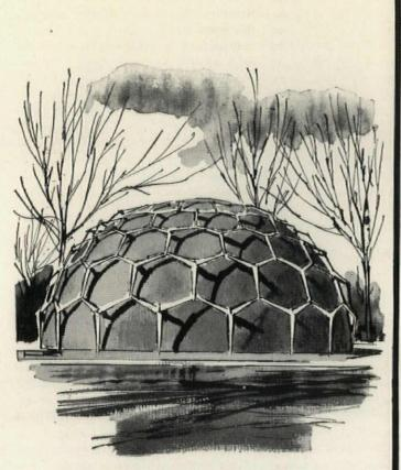
LIGHTWEIGHT, DURABLE, permanently flexible and applied cold — that's the colorful new Butyl roofing system at Longway Planetarium, Flint, Mich., designed by Smith, Hinchman & Grylls Associates, Inc. (Detroit).
