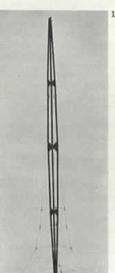
determined range—thus creating what I call a "Reactive System" (1). At each point where the cable meets the ground, an electronic device actuates a pressure pump to bring back the elongation to a fixed value.
