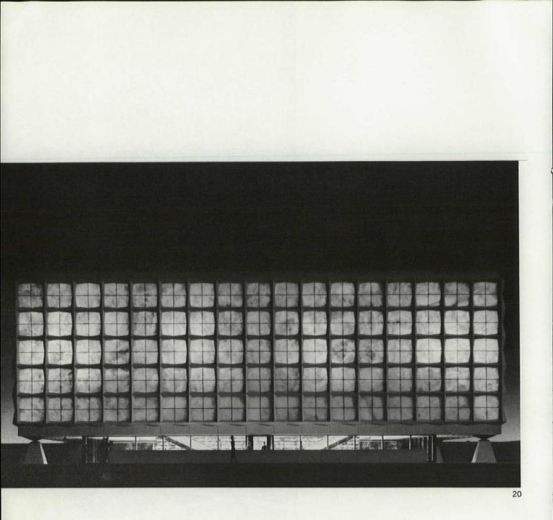
pletely welded to achieve continuity of all joints. Its trusses support marble mullions and sills that frame translucent onyx sash panels.
