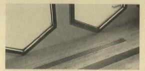
A-E Floor permits flexibility in height of sill around perimeter.
