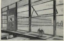
Projected Windows. LUPTON "Master" windows in projected or casement typesused equally well in curtain walls or in masonry construction. Tubular ventilator members for extra rigidity...double weatherstripping, bronze hardware.
