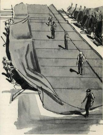
**PROTECTION FOR BUILDING FOUNDATIONS** from both hydrostatic pressure and water infiltration is provided by sheeting of Enjay Butyl rubber. Butyl's high tear strength withstands rough handling on the job site.
