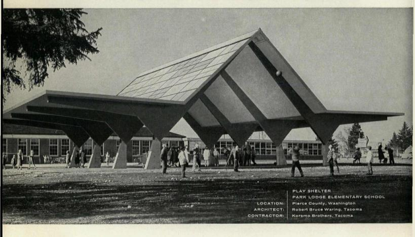
1. PITCHED BEAMS are tapered box beams, with Exterior plywood webs and lumber flanges.
