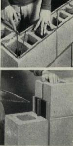
Strength with flexibility-the two basic factors for a repair-free masonry wall are assured by these intelligently engineered companion products. Dur-o-wal reinforcement, top left, increases flexural strength 71 to 261 per cent, depending on weight Dur-o-wal, number of courses, type of mortar. The ready-made neoprene compound flange of Rapid Control Joint, beneath, flexes with the wall, keeps itself sealed tight.
