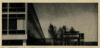
Over 82,000 sq. ft. of FOAMGLAS insulates these glass spandrel panels at the Connecticut General Life Insurance Building, Bloomington, Conn. Fabricated right on the job, FOAMGLAS protects the steel from air and moisture damage while it serves as the backing for the metal flashing that rings the building.
