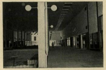
COMPLETELY FIRE-RESISTANT CONSTRUCTION. Masonry fire wall partitions rise unhampered through MACOMBER METAL DECK roof via double framing at roof line. V-LOK columns were embedded in walls. Open web purlins and girders made sprinkler installation easy.
