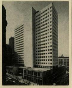
the result of a new construction technique developed by Naramore, Bain, Brady & Johanson, architects of the building, and The Georgia Marble Company. In casting the panels, the marble sections were placed face downward in steel frames, a  $\frac{1}{4}$ " protective coat of white cement mortar was cast against the marble, followed
