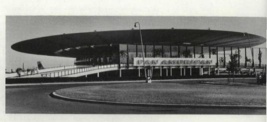
The elliptical roof canopy cantilevers 110 ft to shelter vehicular ramps and plane positions. Outbound passengers enter the concourse through an air curtain (below).
