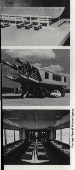
Mobile lounges for the Dulles International Airport (top) can be coupled to the terminal it one end; the other end has folding ramps or access to planes (middle); luxurious inerior (bottom) holds 90 passengers.
