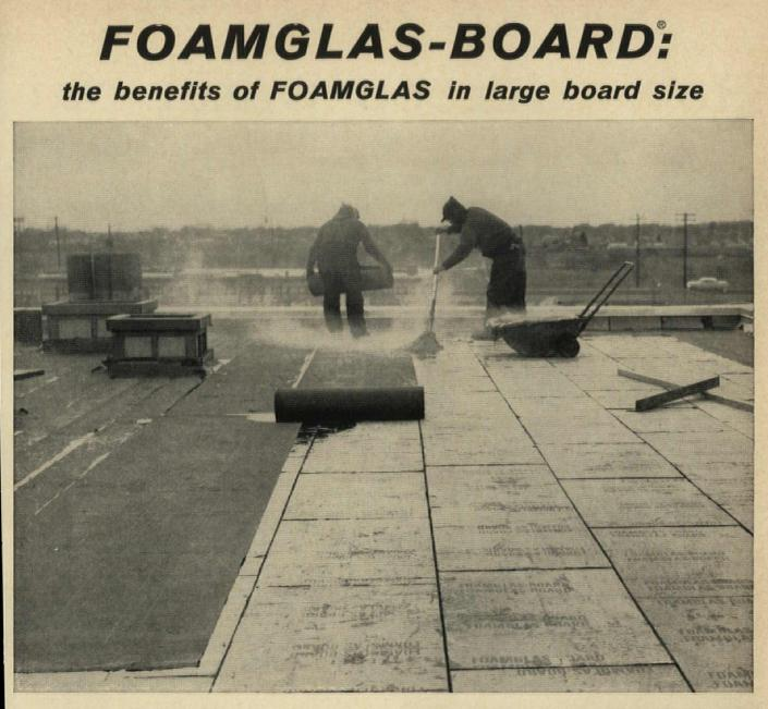
The proven insulation benefits of FOAMGLAS are available now in a special  $2' \ge 4'$  unit, a board size that speeds roofing installation and cuts labor costs.
