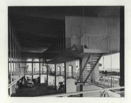
The special "Clipper Lounge" (above) is suspended over the plane positions. The apron is also visible from any part of the main concourse (below). To meet local building requirements, pipes between the canopy and the piers (acrosspage) were substituted for connections originally designed by the architects.
