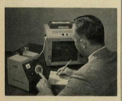
tages is the ease with which offices can prepare their own audio-visual programs. Recording is done on the basic unit, and a 35 mm camera is used to prepare slides. Electronic pulses that automatically change the slides are recorded on the tape along with the prepared commentary.
