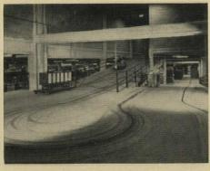
across a bridge to the fifth floor of the store. Similar conveyors have been widely used in railroad and truck freight terminals and in numerous warehousing operations, but this is the first time that such a system moves the entire spectrum of a department store's merchandise.
