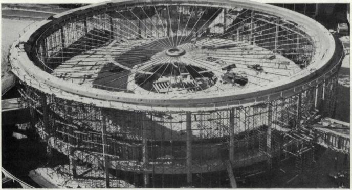
THE AIRPORT RESTAURANT AT CHICAGO'S O'HARE FIELD, shown here under construction. Suspended roof allows maximum seating capacity within framework of economy and beauty. Contractors: E. H. MARHOEFER, JR., COMPANY, Franklin Park, III. Architects-Engineers: C. F. MURPHY ASSOCIATES, Chicago, III. Prestretched galvanized Bridge Strand assemblies by ROEBLING.
