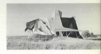
"straight 2 x 4's and 2 x 8's were used to generate the slightly curving walls." A ¼-in. scale model was useful in placing the basic structural members. During assembly of the outside walls, black mineral-coated roll roofing was
