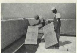
Nothing but FOAMGLAS Roof Insulation gives a building the constant insulating value that results from an inorganic, cellular glass composition. It just can't absorb moisture. And, it's available now in a 1½" thick FOAMGLAS-BOARD PITTSBURGH
