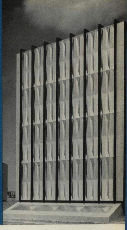
These monumental intake gate structures are new landmarks on the Niagara River. The functional severity of the two 100-foot towers has been softened and humanized by brilliant stainless steel curtain wall envelopes, accentuated by black enameled aluminum columns. The structures were designed by Uhl, Hall and Rich—Engineers and Architects for the N.Y. State Power Authority. Contractor: Merritt-Chapman & Scott Corp.
