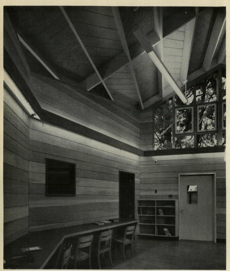
A continuous counter of wood with overhead cove lighting efficiently takes the place of desks. Planked walls, tongue-and-groove ceiling with exposed supports facilitate maintenance—a job performed by students, teachers, and parents in this unique progressive school.
