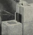
flexibility-the two basic factors for a repair-free masonry wall are assured by these engineered companion products. Dur-o-wal reinforcement, top left, increases flexural strength 71 to 261 per cent, depending on weight Dur-o-wal, number of courses, type of mortar. The ready-made Rapid Control Joint, beneath with its neoprene compound flange flexes with the wall, keeps itself sealed tight. Continued from page 206
