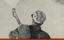
FIRECODE "V" Plaster also sprays directly to corrugated, flat, or cellular steel deck units.
