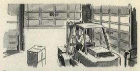
Driver has pulled cord, and "OVERHEAD DOOR" is moving up in Air Express building at Atlanta's new airport. Immediate door operation permits tractors to pull package-laden carts into and out of building, quickly and efficiently, saving many man-hours.
