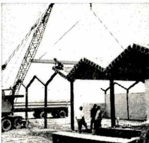
New 8" x 16" Hi-Stress units are fully pre-stressed slabs ( $f_{si}$  175,000 psi) cast in steel forms, with stress-relieved strands tensioned before concrete is poured. Appearance is similar to standard Flexicore slabs which use pretensioned intermediate grade steel bars.
