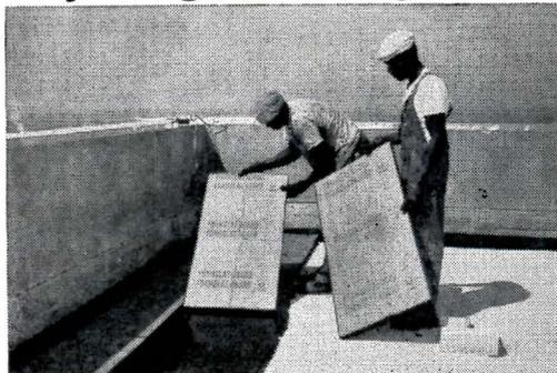
ured insulation permanence. Even if a roof leak should develop, FOAMGLAS will not absorb water, constant insulating value is guaranteed. FOAMGLAS-BOARD's new 1½" thickness in a 2 x 4' board size presents an economical savings in material and in installation costs. FOAMGLAS cuts heating and air conditioning costs, so savings begin with the specification. Write for our Building Insulation Catalog: Pittsburgh Corning Corp., Dept. AB-82, One Gateway Center, Pittsburgh 22, Pa.
