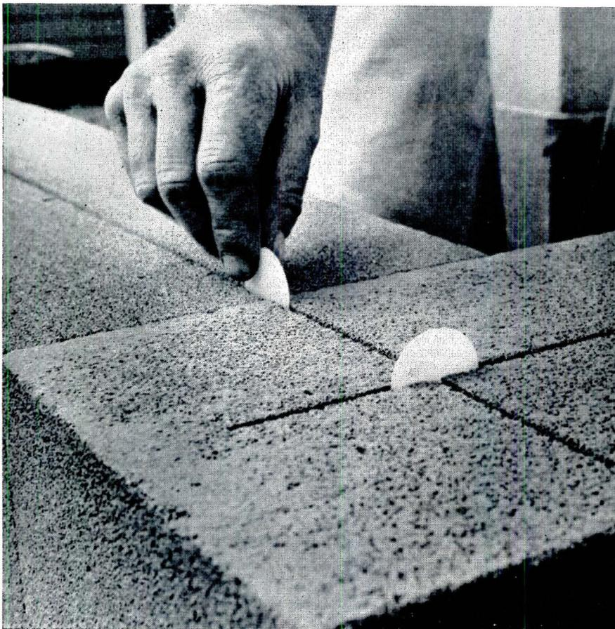
*Report on a new method of joining lightweight-concrete building units, using plastic discs instead of mortar.*
