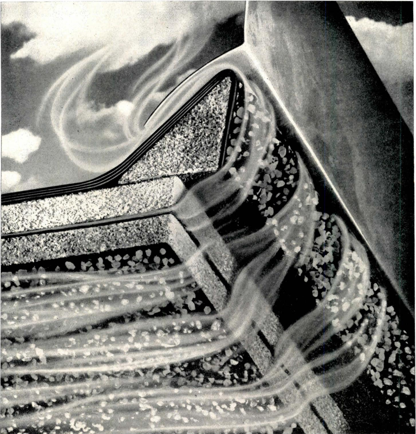
Roofinsul or J-M Fesco Board—is kerfed on all four edges. This provides still another avenue for air and moisture to travel out of the roof assembly through vent spaces at the edges of the roof.
