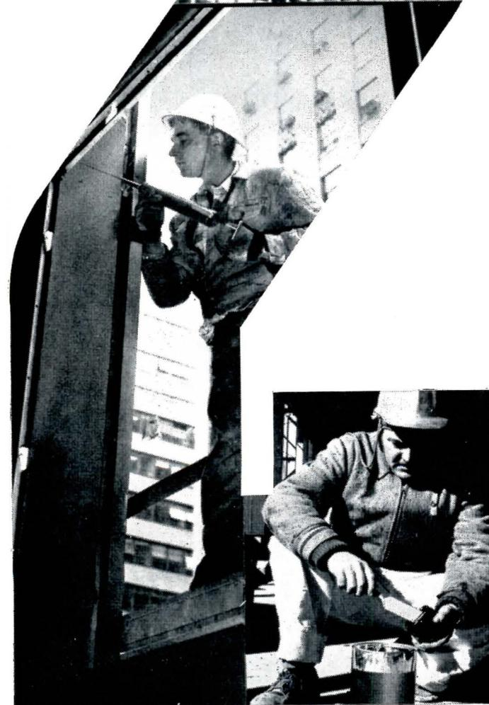
**Satisfying for the architect.** Polysulfide base sealant has been field proven since 1952. History of its successful weatherproofing ability corresponds to the success of the modern curtain wall. It includes application in both dynamic and static joints and service in all kinds of structures and all weather conditions. Quality of the material can be measured against American Standard Specification A116.1. You can specify polysulfide base sealant with an extra measure of certainty.
