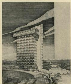
reinforced concrete which will contain stair towers, elevators, and mechanical and electrical equipment. Under the top restaurant and terrace level, cantilever trusses will extend on three sides to support vertical steel tension members from which the lower floors will be suspended. The exterior grill pattern will be incorporated with the ver-*Continued on page 76*
