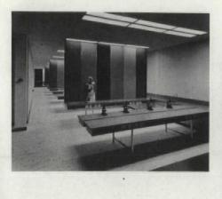
In the classroom block of the Life Science Building (below), ten cross-shaped columns support 19' x 24' structural "capitals" (right) that carry the remainder of the second floor and roof. Precast concrete sunscreens protect the classrooms on the upper floor (left). The windowless, loftlike laboratory spaces (above) are partially divided by asbestos panels finished to double as chalkboards.
