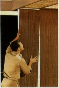
For fast installation, Marlite Random Planks  $(\frac{1}{4''} \times 16'' \times 8')$  are tongued and grooved—assure a better finished job.
