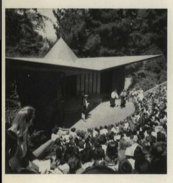
THIS INGENIOUS STAR-SHAPED ROOF demonstrates the remarkable structural forms that can be achieved with plywood. Deceptively simple, the design bears more resemblance to airplane wings than a conventional roof, with interacting plywood and lightweight lumber members forming skeleton and structural skin.
