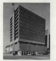
Recent examples of load-bearing exterior walls for office buildings. Massive 23-ft-deep girder, enclosing mechanical room, spans 56-ft column spacing (1). Two-pylon-points of support for each wall truss, spaced 27 ft apart on longitudinal elevation and 54 ft on transverse, define location of core (2). Transition floor, 10 ft deep, supporting bearing-grille wall above, and also enclosing air-conditioning equipment, extends 42 ft between columns (3).
