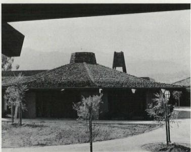
The octagonal science lecture hall building (above) is one of three similar structures on the campus, the special function of which is expressed in their form. In this case, the octagon is divided into three halls (plan at left), separated by common preparation space. The wood-paneled interiors (left) follow the form of the structure. The court in the science group (facing page) features a tower with a Foucault pendulum.
