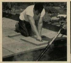
EASY TO CUT (on the average job 30% of insulation must be cut)
