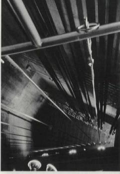
Instead of basement drying racks, a hose drying tower (above) was used to introduce a strong vertical element to the building mass (facing page). Concrete structure is exposed in the apparatus room (right and below), staircases (bottom), and all other parts of the building.
