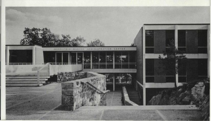
Precast exposed-aggregate concrete columns and spandrel panels establish a light-colored framework for the typical wall (photo below), within which are set darker materials—gray glass, purplish slate, and red brick. The architect's original choice of "brownish" brick, to harmonize with the slate, was changed to red brick for the sake of conformity. The penthouse offices have been accentuated by a vaulted concrete roof.
