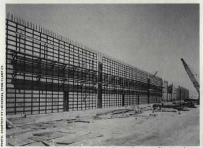
Gang-use of prefab forms for extremely long walls of new filtration plant.
