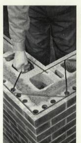
Strength with flexibility-the two basic factors for a repair-free composite wall are assured by Dur-o-wal. Around corners, that is, as well as in the straight stretches. Positive, continuous reinforcement of corners is easy when formed on the job -even easier with prefabricated Dur-o-wal corners such as shown in this picture.
