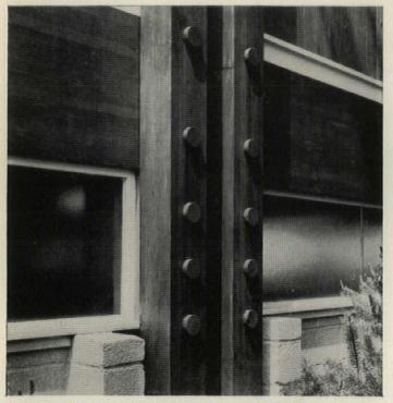
A close-up of the club's laminated posts shows off the inherent strength of wood in fist-sized peg fastenings. This grass-high view also illustrates wood's compatibility with the barest forms of glass and concrete.
