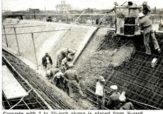
Concrete with 2 to  $2\frac{1}{2}$ -inch slump is placed from  $\frac{3}{2}$ -yard bucket on forms for folded plate roof. Roof is made up of 8 V-sections 26 ft wide and  $11\frac{1}{2}$  ft deep, each post-tensioned with 12 tendons.
