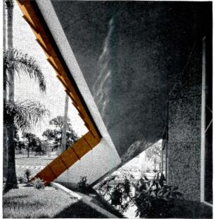
FASCIA was prefabricated in the sheet metal contractor's shop in 4' sections with a 2" standing seam.
