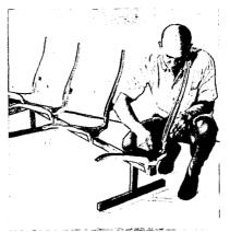
Assembly: frames secured to tee beam.
