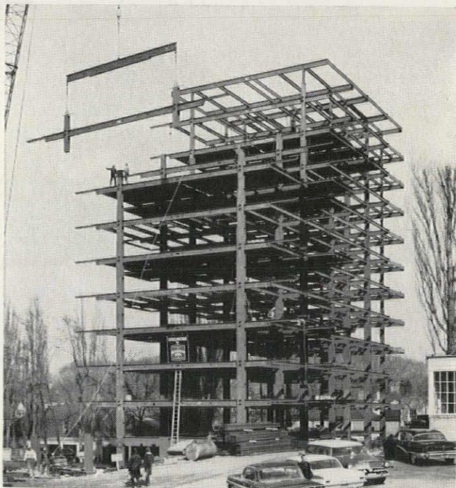
Topping out a section of the steelwork. It took just 17 working days to erect the complete 775-ton frame.
