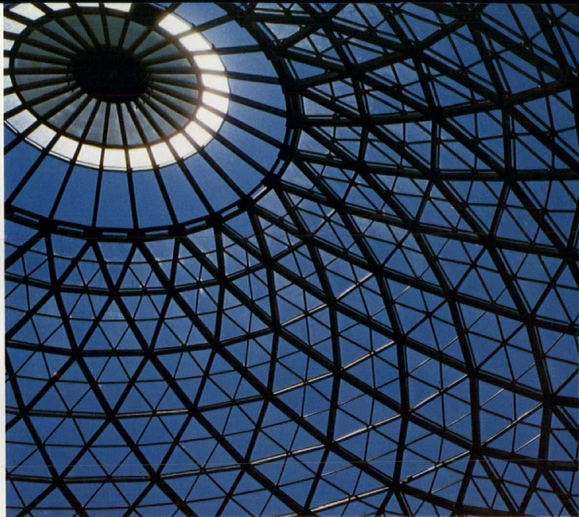
Close-up detail of complete skylight section. Rugged, Polished Misco wire glass combines the utmost in safety with modern beauty . . . affords approved yet inconspicuous fire and breakage protection wherever installed.
