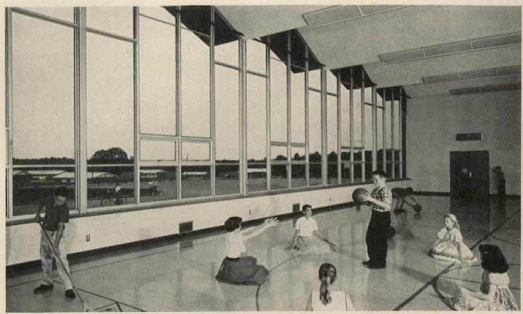
Window wall in gymnasium is glazed with Parallel-O-Grey Plate Glass that has been heat tempered for extra strength.
