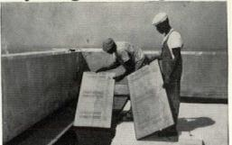
FOAMGLAS will not absorb water, constant insulating value is guaranteed. FOAMGLAS-BOARD's new 11/2" thickness in a 2 x 4' board size presents an PITTSBURGH economical savings in material and in installation costs. FOAMGLAS cuts heating and air conditioning costs, so savings begin with the specification. Write for our Building Insulation Catalog: Pittsburgh Corning Corp., Dept. AB-23, One Gateway Center, Pittsburgh 22, Pa.
