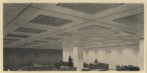
One of the unique features of the Bankers Trust Building which recently opened in New York [p. 44, JANUARY 1963 P/A] is its ceiling lighting system. Designed by General Electric with Consultant Richard Kelly, the units consist of a plastic grid louver with aluminized reflecting surfaces that are parabolic in shape. This system creates a low-brightness lighting in which the light is directed downward instead of into the eye. Thus, even if an interior is completely
