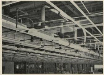
During installation view of two outside (perimeter) rows of troffers. On the outer row, each troffer has an air connection; on the inner row, every other troffer is connected.
