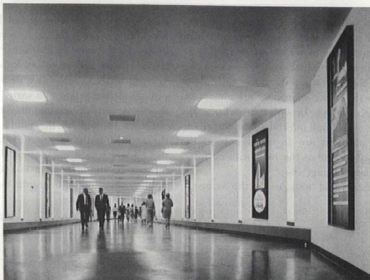
floors there are of concrete, ground to expose the aggregate.
