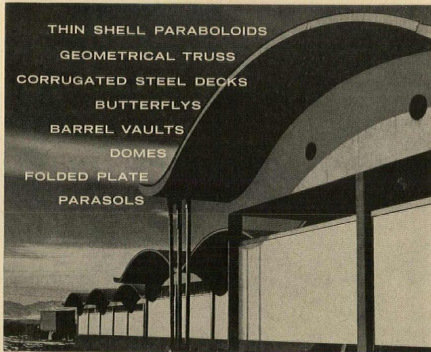
**A.** Permalite insulating concrete, with 'k' factors from 0.77 to 0.51, is easily applied to *any* shape roof deck with standard equipment. Weighs only 3½ to 6¾ lbs/sq. ft., 2" thick, with compressive strengths to 500 psi. Permanent. Rot-proof. Fire-proof.
