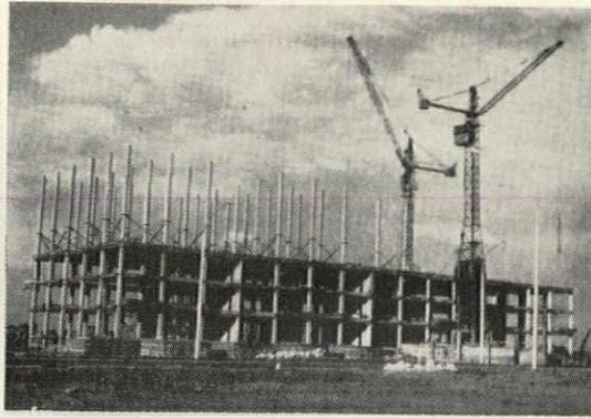
Large prefabricated units in Polish apartments; and prestressed-concrete columns in a Yugoslavian system.
