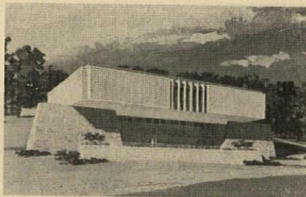
& Miller of North Allentown, the building will utilize a campus hillside as its site, causing the main entrance to be approached via a bridge over a dry moat into the upper story reading and information areas. This floor will be cantilevered at the rear (as shown) over the stone retaining walls enclosing the lower areas. Library is the first of three new buildings in the college's 10-year development program.
