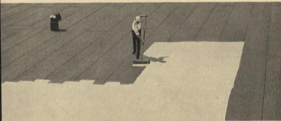
**Last-O-Lume**, the reflective surface finish, is an elastomer-based coating, formulated for compatibility with all Last-O-Roof membranes and adhesives. It's available in durable aluminum, white and metallic pastel colors to harmonize with any building design. The highly reflective surface will aid in lowering roof and interior temperatures.
