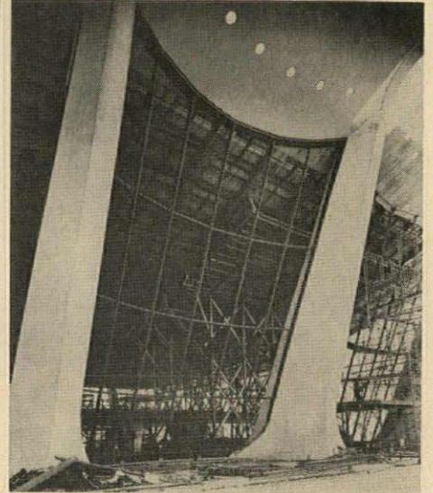
columns in the terminal is approximately 40' wide by 50' high. Neoprene gaskets seal the joints between the mullions and the 1/2" plate glass and the steel framework. Revere Copper & Brass, Inc., 230 Park Ave., New York 17, N.Y.
