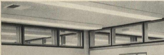
Centrally conditioned air is ducted to ceiling diffusers. High window strips give a feeling of spaciousness and eliminate distractions. Refrigeration is provided by two Carrier Automatic Absorption Machines powered by low-pressure steam which also supplies heating.
