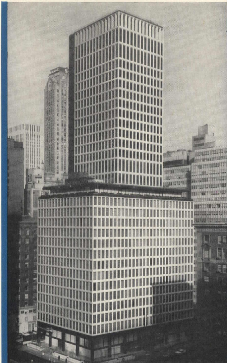
Erected individually, the precast units were quickly hoisted, bolted in place and caulked.
