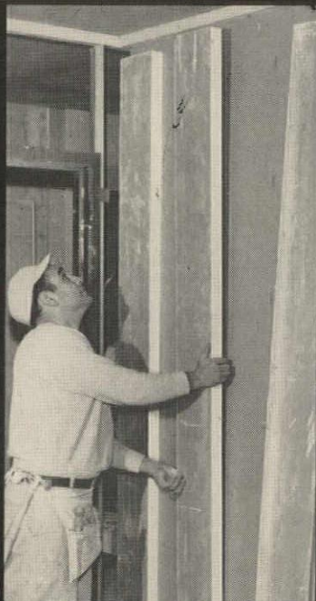
2. Apply adhesive-coated gypsum studs
