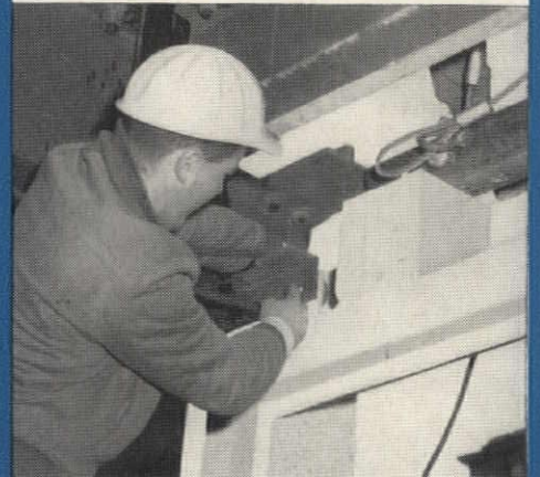
Erected individually, the precast units were quickly hoisted, bolted in place and caulked.
