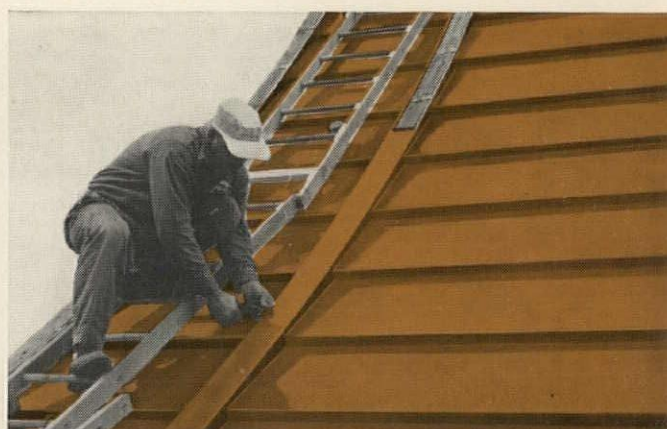
(above) HERE YOU SEE batten covers being affixed. (below) ROOF DETAIL showing method of forming roof pans, with pans and battens in place.
