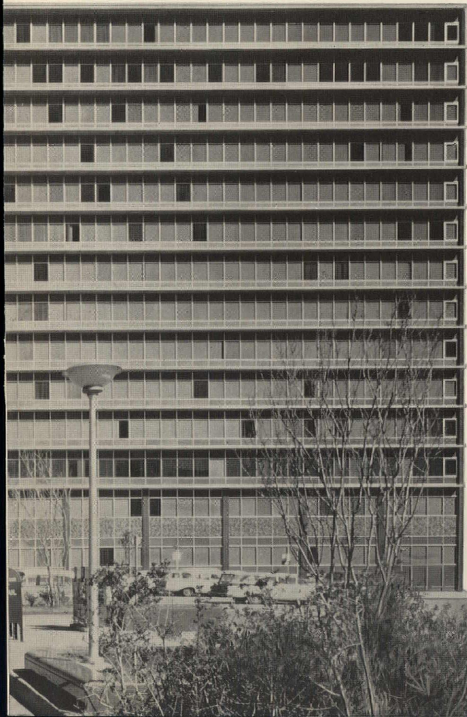
Detail photograph of Pittco 82-X Curtain Wall. Clean, crisp members show no visible fasteners—accept glass and mosaic spandrel panels without modification. Note distinctive reflective quality of PPG SOLARGRAY Plate Glass.
