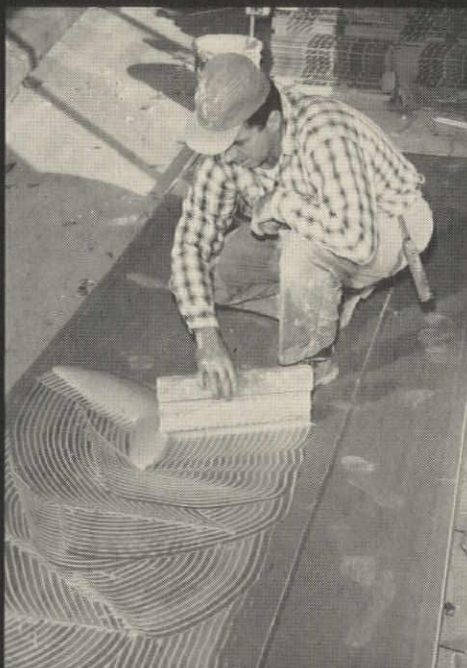
D. Apply adhesive to back of gypsum face layer
