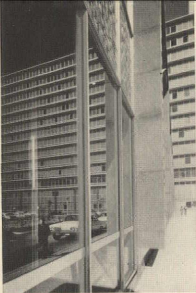
Detail photograph of Pittco 82-X Curtain Wall. Clean, crisp members show no visible fasteners—accept glass and mosaic spandrel panels without modification. Note distinctive reflective quality of PPG SOLARGRAY Plate Glass.
