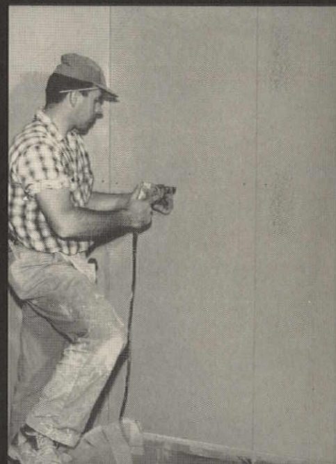
E. Screw face panels to gypsum coreboard on each side of double-wall partitions
