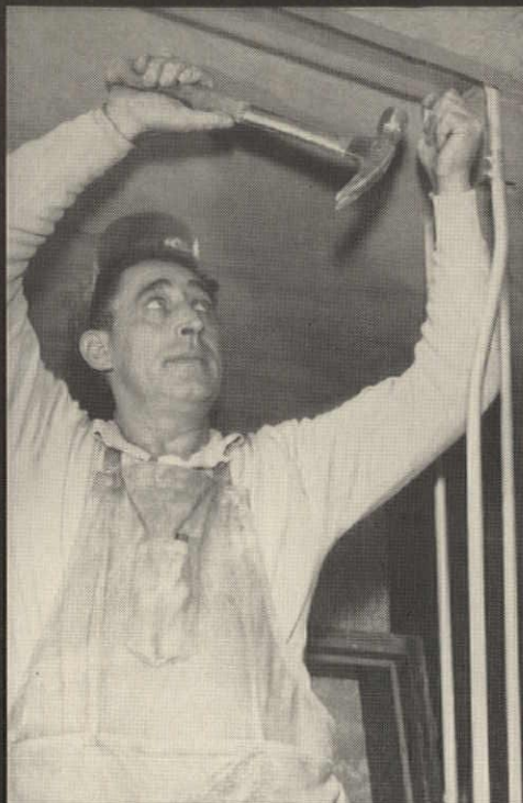
A. Install metal floor and ceiling runners
