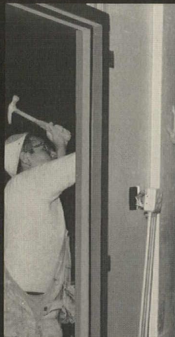
3. Secure gypsum studs with nails or screws
