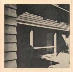
tion and durability. One side of cedar bevel siding is smooth-surfaced and the reverse side is saw-textured. Brochure also includes grades, sizes, application and finishing procedures. Western Red Cedar Lumber Assn., 4403 White-Henry-Stuart Bldg., Seattle 1, Wash.
