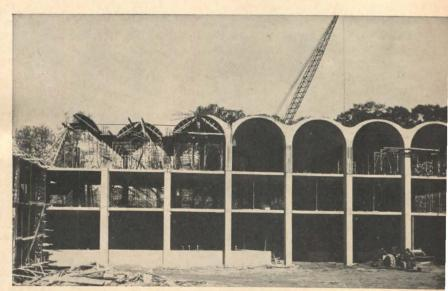
Beams, columns and barrel-arched roof are all reinforced concrete, cast in place.
