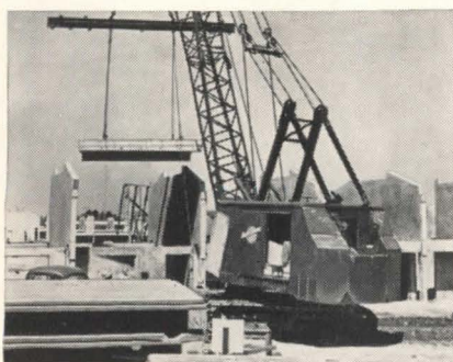
A second floor slab being lowered into place. Supporting beams are cast as an integral part of the slab. Connections are made with weld plates cast in the units.
