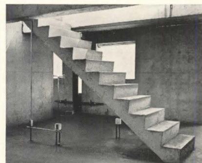
Precast stairs connect the first and second floor of each dwelling unit. Stair forms are positioned on a graded embankment and ready mix trucks dump concrete from the top.
