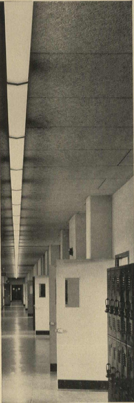
Intermittent noise and confusion in busy corridors is controlled by sound-absorbing Tectum.
