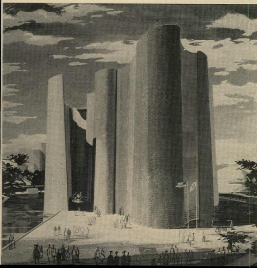
Three asymmetrical cones distinguish roof of Sierra Leone Pavilion; forms give circular feel to a rectangular pavilion. Architect: Costas Machlourarides; Associate: Ransford Jarrett-Yaskey.
