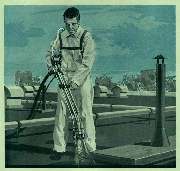
No other single method of application has ever caught on so fast as the Flintkote MONOFORM Roofing System. Using the versatile Flintkote SEALZIT® roofing gun, special Monoform compounds are applied simultaneously with chopped glass fiber reinforcement. It replaces conventional roofing, re-roofing and maintenance methods of building up a roof layer by layer with felt and "hot mopped" asphalt. Millions of square feet of Monoform roofing have
