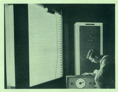
Reduced cost of both light and total energy systems in commercial buildings have long been sought in the electric field (pp. 118–121, MARCH 1953 P/A). In order to reduce these costs, a combination high efficiency converter and ballast has recently been developed to convert 60-cycle fluorescent lighting systems to 3000 cycles. Converter utilizes electric power at efficiency rate of 91 per cent as compared to that of 85 per cent for 60-cycle systems.
