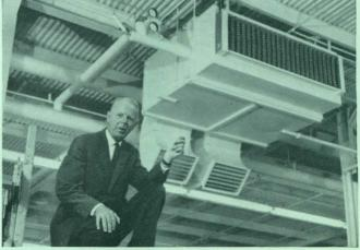
**COMBINATION ELECTRIC UNITS** suspended from roof provide air conditioning in summer and have built-in resistance coils for winter heat. Chief Engineer Russell Bush points out their compactness.
