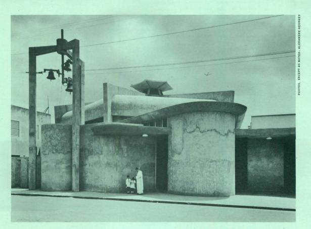
and for local construction methods. An earlier design, with Dr. August E. Komendant as engineer, was for precast concrete (see his article, "Concrete Technology," OCTOBER 1960 P/A), but costs forced the change to cast-in-place.
