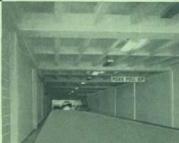
Interior view shows double tee and concrete masonry construction.
