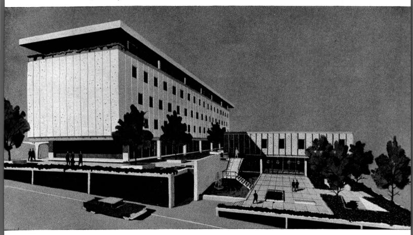
Everett Associates, Architect-Engineer, investigated both reinforced concrete and structural steel for the framing material . . . then chose <u>steel</u>, when steel proved more adaptable, more economical.
