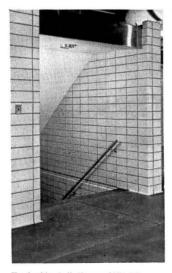
Typical installations of Vitritile are shown in passageway and stairwell. Nominal face size of "6T" series Vitritile (at right) is  $5\frac{1}{3}$ " x 12"—in 2", 4", 6", and 8" thicknesses.
