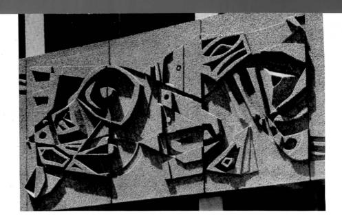
Exposed-aggregate, sculptured panels are at the stage of development where they can be rapidly produced at prices comparable to other building materials. Casting procedures and other steps in the process of creating these panels are discussed.
