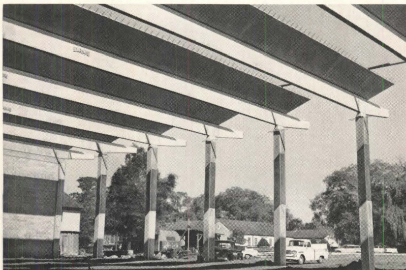
Eight prestressed Y beams are set in place on 16' centers as the first step in roof construction. Each beam measures 105' long and 8' wide.
