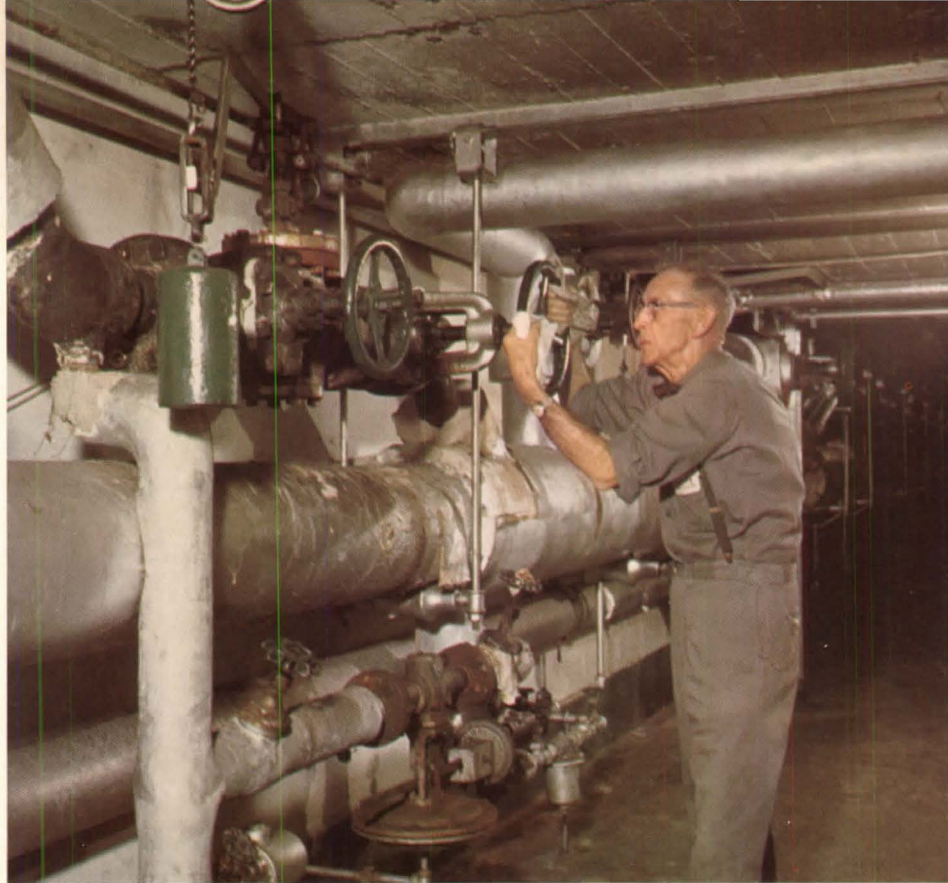
Before: Turning on the heat at Harvard's North Yard buildings once meant daily 2-hour tours through steam tunnels for Isaac H. Larew, engineer, and a crew of associates.
