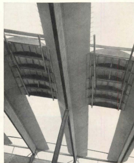
To complete the interesting form of the roof, 8' wide parabolic arches are poured in-place between the beams.
