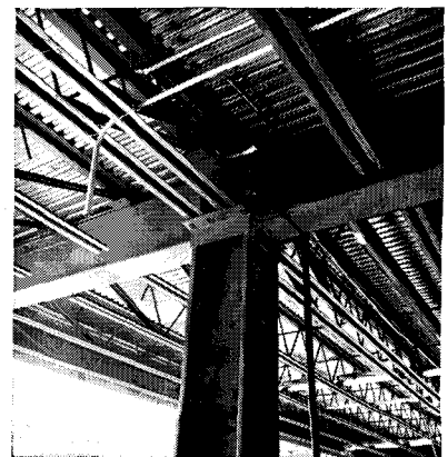
Steel joists allow pipe, conduit, and ductwork to be run in any direction.
