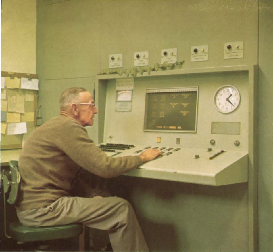
After: Seated at this Honeywell console, Larew now can supervise systems in 67 buildings of Harvard's North Yard, operating 32 steam valves, 42 fans, up to ½ mile away.
