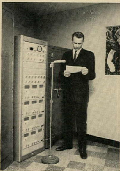
Each floor has its own Webster sound control center. Components to provide additional sound services can be added as required.
