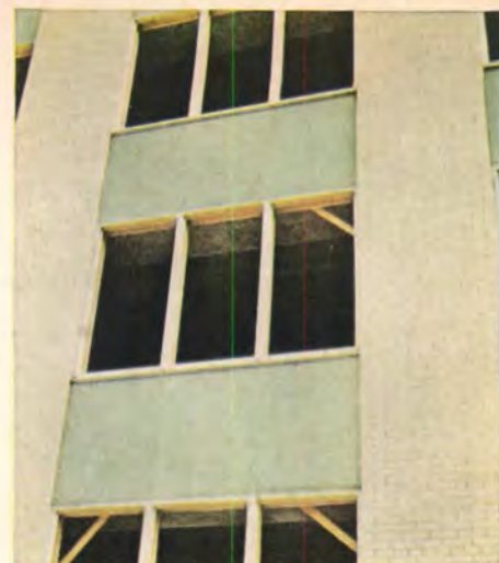
Spandrels of Surf Green Colorlith with masonry back-up.
