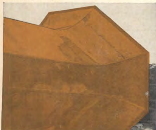
COPPER SPIRE for Church of the Open Door, Muskegon, Mich. It was fabricated from 5,000 lbs. of 16 oz. Cold Rolled Revere Copper by LIVINGSTON SHEET METAL CO., Muskegon. Spire is 81 feet high and 19 feet in diameter at the base. Revere Distributor: CENTRAL STEEL AND WIRE COMPANY, Chicago, Ill.
