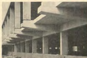
Lateral beams at second floor cantilever 7'-3".
