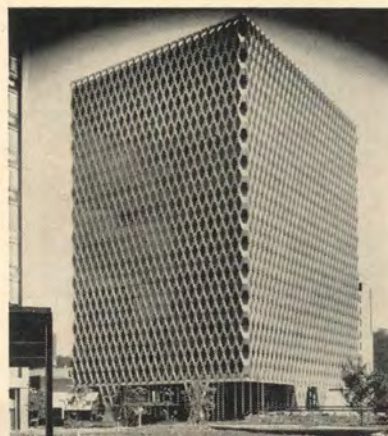
Stainless Rigid-tex Metal Pattern #2-WL provides visual flatness plus cost savings over other metals in the 13-story IBM Building, Gateway Center, Pittsburgh. Architects: Curtis & Davis. Stainless Fabricators: Limbach Company.
