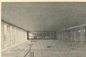
Long span Hi-Stress ceiling before partitions installed.
