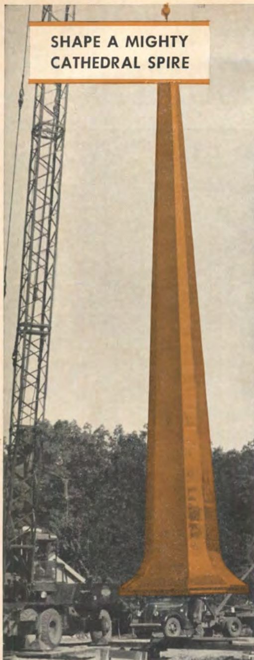
COPPER SPIRE for Church of the Open Door, Muskegon, Mich. It was fabricated from 5,000 lbs. of 16 oz. Cold Rolled Revere Copper by LIVINGSTON SHEET METAL CO., Muskegon. Spire is 81 feet high and 19 feet in diameter at the base. Revere Distributor: CENTRAL STEEL AND WIRE COMPANY, Chicago, Ill.
