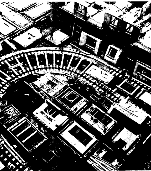
22 Crane demolds and places units
