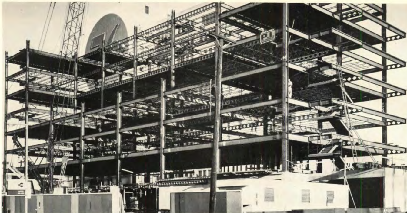
Sheffield H-Series Joists in floors of Doric Motor Hotel
