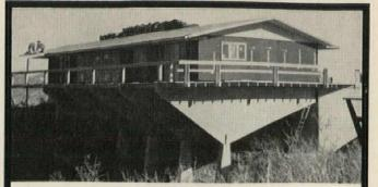
HILLSIDE LOTS - This home has a substructure of five inverted wood girders, each composed of three Sanford trusses boxed in plywood, mounted on concrete piers. Savings in labor, materials and site grading enabled the architect to use this steeply-sloped lot efficiently.
