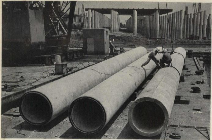
54-inch-diameter prestressed concrete piles on barge, ready to be spotted for driving.
