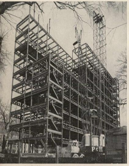
Castellated beams are Bethlehem 16-in. wide-flange "expanded" to 21 in. to save weight and provide additional strength for wind bracing. Bethlehem supplied 183 tons of H-piles, as well as 600 tons of structurals. General Contractor: J. Migliore Construction Co., Buffalo. Steel Fabricator and Erector: Rebco Steel Corp., Niagara Falls, N. Y.
