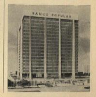
and serve as conduction tubes for air conditioning. Banco Popular Center, as it will be known, rests on a mat foundation that in turn is supported by a total of 10 miles of concrete pilings. Its most prominent feature-the name in story-high letters, capping the building-is like an admission that the design is bland enough to make a label obligatory. Engineers for the project are Lev Zetlin & Associates of New York and Dinos & Vafi of San Juan.
