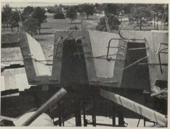
formed by placement of top units on identical inverted bottom units, demanding close tolerances. Protruding re-bars will be anchored into the poured concrete compression ring.
