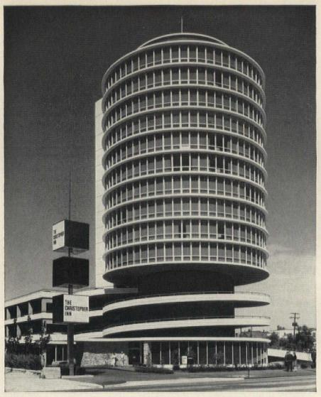
The Christopher Inn, Columbus, Ohio's first downtown motor hotel, is a striking 16-level circular cantilevered tower. The Inn has 140 rooms, beginning on the fifth level. Parking for 110 cars is provided on second, third and fourth levels. High speed elevators provide rapid service to all floors. Central core houses utility shafts and stairwell. To rear of tower is a 5-story rectangular building with meeting and dining room accommodations for up to 500 people.
