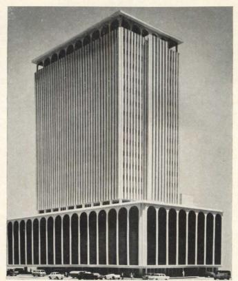
Model of 22-story Exchange National Bank Building shows ground floor for banking facilities, six-story parking garage, and office tower section with floors designed for composite action.
