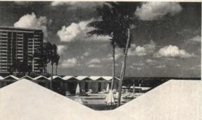
A single ply of roofing gives long-lasting whiteness to the prominent, folded-plate roof of this hotel cabana. The surface of Du Pont TEDLAR\* PVF film will remain a brilliant white, even after years of exposure. The roofing is Ruberoid T/NA 200† with TEDLAR. T/NA 200 is easily installed with conventional roofing techniques. It weighs less than conventional built-up roofing, and it can fit roofs of unusual contour and of any slope.
