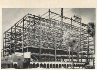
34% of the 3,200 tons of structural members supplied by Bethlehem is V50 and V55 high-strength steels. Field connections were welded and high-strength-bolted; shop connections were welded (V Steels are readily weldable).
