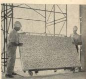
Prefab panels of ceramic tile facing are used in 14-story Banco de Ponce office building in San Juan, Puerto Rico. Mosaic panel walls are 66 per cent lighter than precast materials and weigh 10 to 16 psf, depending on surfacing used. Panel is about one-third the weight of reinforced concrete and has good strength-toweight ratio. Panels meet requirements for Class A construction by New York City
