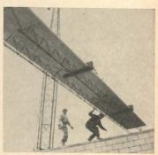
including built-up roof, ranging between 25.5 psf and 28.4 psf, depending on span. Joists (according to Steel Joist Institute specs) are placed 2' for both floor and roof slabs. At present, distribution of these slab units is limited to within 200 miles of Pennsylvania plant. Clearspan Inc., Catasauqua, Pa. On Readers' Service Card, Circle 104
