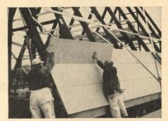
T & G panels, 2' x 8', serve as decking and sidewall for this A-frame with 48'' o.c. spans. Interior surface can be factory-coated in white, beige or special color to order-with vapor barrier and vinyl film or white kraft surface.
