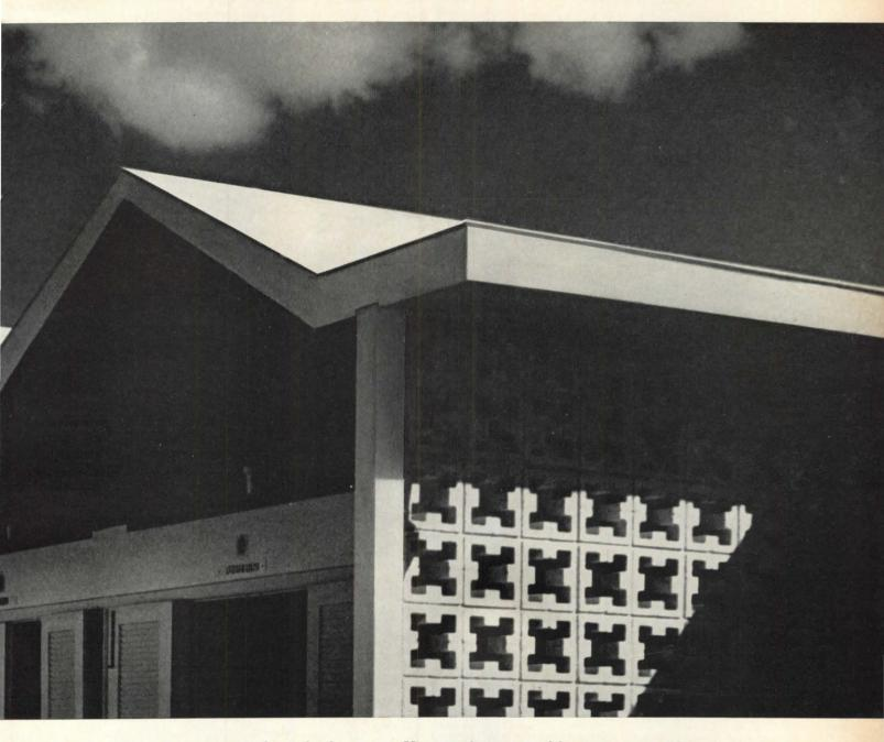
half the solar absorptance of crushed stone or marble), which lowers underroof temperatures and air-conditioning loads.
