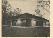
Shown above are photos of a mock-up designed and erected by the School Construction Systems Development (SCSD) project at Stanford University -a combined effort of the School Planning Laboratory at Stanford and the University of California's Department of Architecture at Berkeley. Ezra Ehrenkrantz was the architect for the completed school mockup, which incorporates a prefab roof system. The project was sponsored by a \$257,000 grant from the Ford Foundation's Educational Facilities Laboratory.
