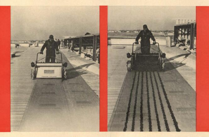
**Pyro-Kure is the permanently noncombustible vapor barrier** that makes Class I Roof Construction on metal decks safer, easier and less costly: Pyro-Kure has twice the vapor resistance of vinyl film, resists abrasion, tears and puncturing during application, and is approved for use with regular asphalt.
