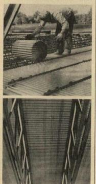
composite joist system has 20 per cent less deflection, produces savings in cost of steel because top chords need only be designed for the basic support of construction loads, and reduces amount of bridging or lateral support. Laclede Steel Co., Arcade Bldg., St. Louis, Mo.
