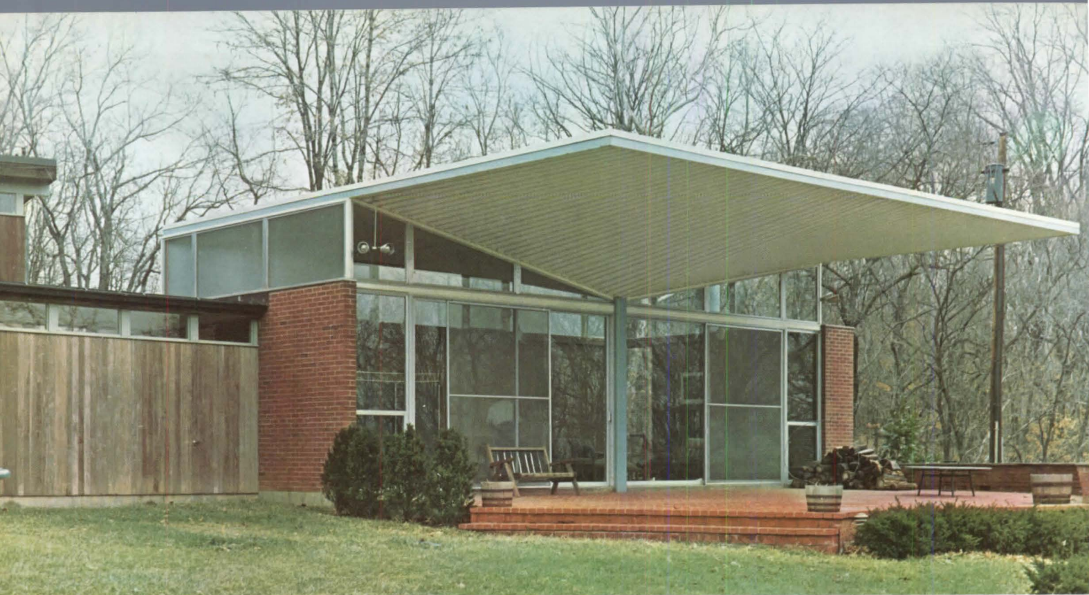
Private home. A striking playroom and a terrace addition were built using a hyperbolic paraboloid roof. Two panels cover the playroom, and two panels cover the terrace.
