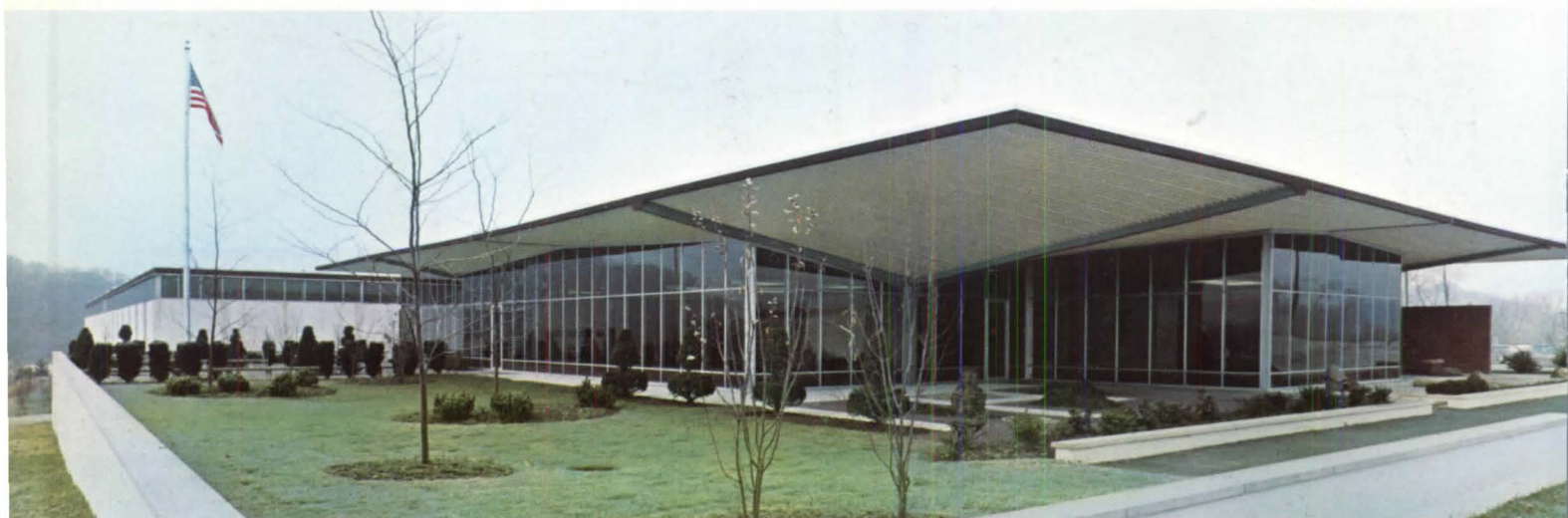
Johnson and Hardin Printing Plant (also cover photo). Hyperbolic paraboloids of two thicknesses of 1\frac{1}{2} " deck form the office building roof, 106'-8" x 133'-4" overall (over 14,000 sq. ft.), supported by but four columns. Each bay is 53'-4" x 66'-8". In the bindery, the exterior bays consist of 40' x 66'-2" umbrellas, articulated by surrounding one foot wide ribs. The bindery is 100' x 100'.
