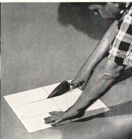
Perfect joint alignment assured, tabs cut easily with a trowel.
