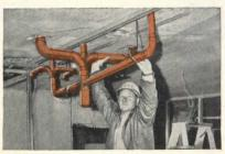
A pre-assembled unit of copper soil, waste and vent branches is easily positioned. Supported by preplaced hangers, it is ready for joining to rest of system. Note the space that is saved by this compact assembly of copper tube and solder-joint fittings.
