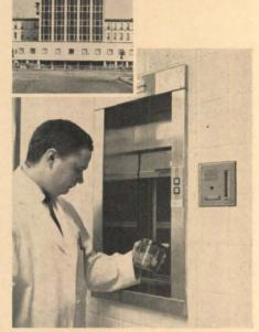
At St. Francis Hospital, Evanston, Illinois, 7 dumbwaiters in combination with an inter com system are being used to increase hospital efficiency. With a new addition increasing their capacity from 385 to 516 beds, the new system was introduced to relieve the added burden on their staff.
