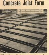
"Unadome" is a system for forming concrete joists in standard widths and modular lengths. Flanged on all four sides, the formwork units can be moved by compressed air. Pamphlet gives sizes, weights, and basic layouts for concrete joist floor construction. 6 pages. Grid Flat Slab Corp., 145 Freeport St., Boston, Mass. On Readers' Service Card, Circle 220
