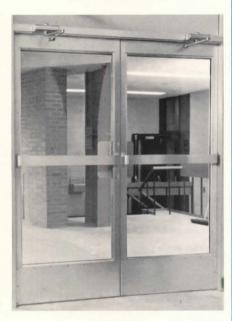
GYMNASIUM ENTRANCE doors with Norton Series 1600 Closers top-jamb mounted. These closers could have been installed just as easily regular arm or parallel arm.
