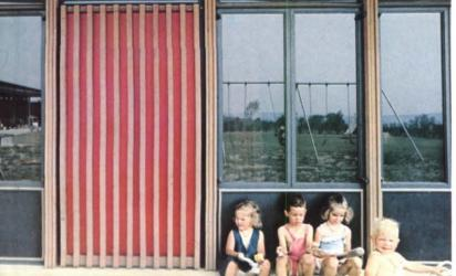
**Double-duty doors.** One louvered door hung from another gives full closet a permits free flow of air to exhaust ducts concealed in closet ceiling. Novodors<sup>®</sup> heavy-duty stile construction were factory pre-machined for hardware and prefinished with solid color Permagard<sup>®</sup>. St. Vincent's Infant Home, Towson, M
