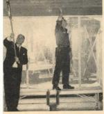
I-Strip" secures radiantng cables to ceiling withusing nails or screws. s are cemented to ceiling posite ends of a room, and ntinuous heating cable is between the strips. ufacturer claims Ceil-Strip es cost of installing radiceiling cables. Extrud-Oc, Inc., 316 Meyer Rd., enville, Illinois. eaders' Service Card, Circle 101
