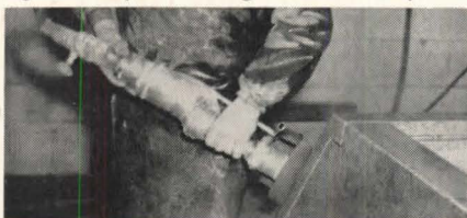
After stripping forms, workmen grind surface of granite-faced precast concrete panels.
