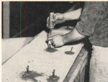
Steel bolts embedded in back of granite facing panels anchor them to concrete.
