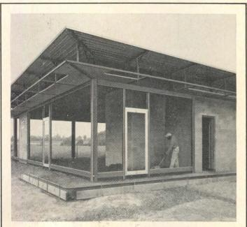
**4.** Square and rectangular tubing serves both as structural components and architectural members. For example, no additional window framing around glass is required. High strength-to-weight ratio makes Republic Structural Tubing an ideal structural material for low-rise construction.
