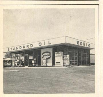
**5.** Finished service station has pleasing appearance and was economically erected with Republic ELECTRUNITE Structural Steel Tubing.
