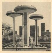
The era of the old oaken water tower is rapidly passing out of style, as is illustrated by this portfolio of new design ideas for water storage in steel by Peter Muller-Munk, an industrial designer from Pittsburgh. Included are such unexpected projects as an elevated tank with an observation roof, and a ground-storage tank ringed at the base by shops and topped by a skating rink. The three basic types shown-ground storage, standpipe, and elevated
