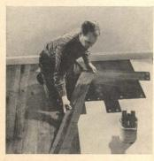
Hardwood veneer, laminated between clear vinyl top sheet and aluminum-vinyl-asbestos backing, makes a flooring only .08" thick. "True Wood" installs like vinyl tile and is said to be tough, durable, and resistant to common stains; it can therefore be used in kitchens and bathrooms. Walnut, cherry, and oak are the standard woods, available in random widths, in squares, and in special parquet and herringbone patterns. Wood-Mosaic Corp., 5000 Crittenden Dr., Louisville, Ky.
