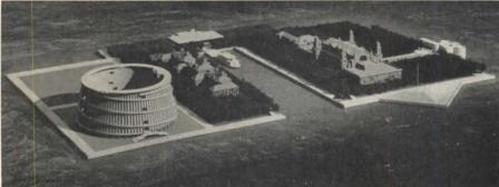
The cone will be spiraled within and without by 8-ft-wide ramps ascending to viewing platforms at various points of the structure. Johnson hopes to have plaques bearing the names of the immigrants who entered the U.S. through Ellis Island mounted between the vertical, prestressed concrete ribs of the building. A 100-ft-diameter pool will be located at the interior of the great court.
