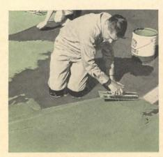
Quick, easy application. Just prime the surface, add catalyst to Traffic Topping, mix and trowel on. No expensive equipment needed. Only one coat is usually required, so application costs are low.
