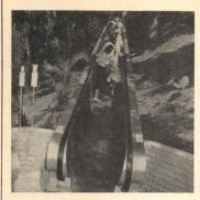
Moving sidewalks or ramps give smoother ride by using belting that requires no center support. A 1"-thick belting is stiffened laterally with wires and rides on rollers that extend only 4" on both sides. Balustrades are either stainless steel or stainless steel and glass. Installation shown is at San Diego Zoo. Stephens-Adamson Manufacturing Co., Transportation Equipment Div., Aurora, III. 60507.
