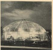
Dome, barrel-vault, pyramid and other types of transparent overhead structures are detailed and specified in two illustrated brochures: "Glazed Enclosures and Skylights" and "Glazed Enclosures and Greenhouses." Domes are built with tubular aluminum framing, thermoformed cast acrylic panels, and aluminum connections that eliminate exposed clips, lugs and bolts. Ickes-Braun Glasshouses, Inc., 1733 N. Western Ave., Chicago, Ill. 60647. On Readers' Service Card, Circle 208
