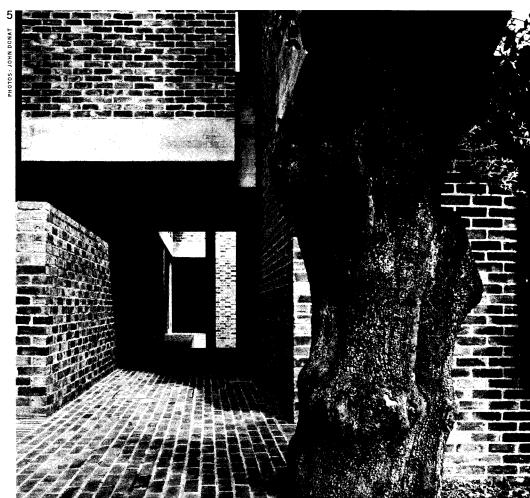
Attention to brick and concrete details is seen in (1) downspouts, which cause water to become coursing part of movement pattern; (2) diagonal pattern of court floor, giving sense of movement across space; (3) slit windows, allowing just enough horizontal light into library and meeting room; (4) interconnecting bridges, which can be used for outdoor theatricals, sunbathing; (5) "pull" of entranceway under low element to lighter, more open areas beyond.
