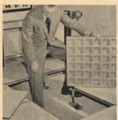
All-steel floor system for rooms requiring underfloor access and plenums comprises 2' x 2' standard panels and adjustable-height pedestals. A stringer system for increasing lateral stability is also manufactured. Brochure contains cutaway views, installation details and specifications. 8 pages. Tate Engineering, Inc., 516 S. Eutaw St., Baltimore, Md. 21201.
