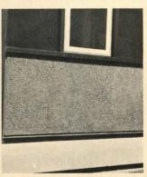
Exposed aggregate concrete, bonded to foamed insulation
