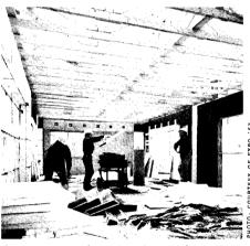
Contractor insulates interiors under a temporary roof, then hoists boxes into place.
