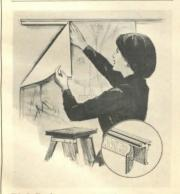
Vel-Strips are Velcro tapes mounted on rigid vinyl strips. When pressed together, the two tapes seal tightly and will support as much as 5 lb shear strength pressure per sq in. The rigid strips, designed for carpet installations, door and wall panels, furniture and drapery installations, and industrial uses, as well as for aircraft interiors and uphol-
