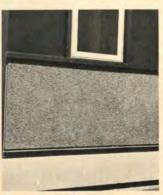
Exposed aggregate concrete, bonded to foamed insulation
