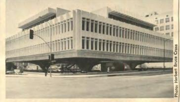
GLENDALE, CALIF. Probably the most striking aspects of the recently completed Municipal Services Building here are the four massively spreading pylons that hold it 21' above street level. At the same time, this stiltlike arrangement merely lets a passer-by see beneath the building to parking lots and streets beyond. The landscaped interior courtyard, which, with its
