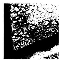
Corner of panel (top) can be expected to fall off when reinforcing fabric exposed in crack oxidizes. Corner may have been cracked during installation of panel, but deepening of crack results from weathering and mortar failure. Sandy matrix (center) provides poor adhesion for aggregate, and cracks will admit water, which will freeze and widen cracks. Stress-cracking pattern (bottom) of small cracks joining large cracks, leave ½-in.-dia. voids where aggregate fell out.
