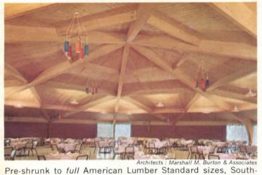
ern Pine provides stability and precision essential to engineered construction, as in this country club. Standard grades can be utilized for cantilevered and continuous members without special grading.
