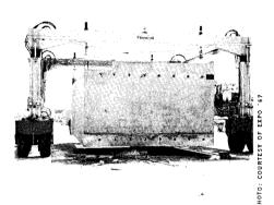
Custom-designed lifting equipment moves precast boxes into storage yard.
