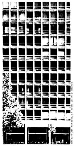
"... a structural grid ... rigid in its own plane ... dense enough to assume the plastic qualities of a bearing wall."
