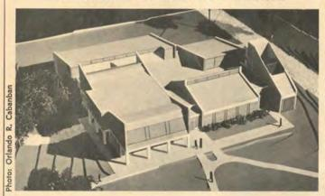
JACKSONVILLE, ILL. This fall, construction will begin on Illinois College's Student Center, a multipurpose complex that uses every trick in the book. Vaulted laminated wood beams and deck, clerestory, floor-to-ceiling and vertical slot windows, varying roof heights, sloped parapets, and
