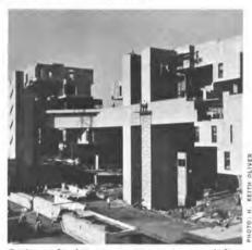
Stair and elevator towers support girders bracing building against horizontal forces.
