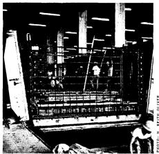
Hydraulically-operated steel walls form 80-ton concrete boxes at on-site plant.
