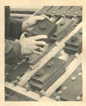
Bolts to match weathering steel are now available. Maintenance-free "Weather-R" bolts with "built-in corrosion resistance" have been developed for use with manufacturer's "Mayari R" weathering steel, which forms a dark brown textured finish after long exposure. High-strength fasteners meet mechanical and dimensional requirements of ASTM specification A325. Bethlehem Steel Corp., Bethlehem, Pa.
