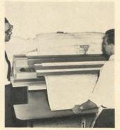
Combination developer and printer for reproducing drawings has added the ammonia system to the developer section. Ammonia control container needs no venting and, after being filled, the "Diazo-Jet" may be left on all day with no further attention. Care and operation of the
