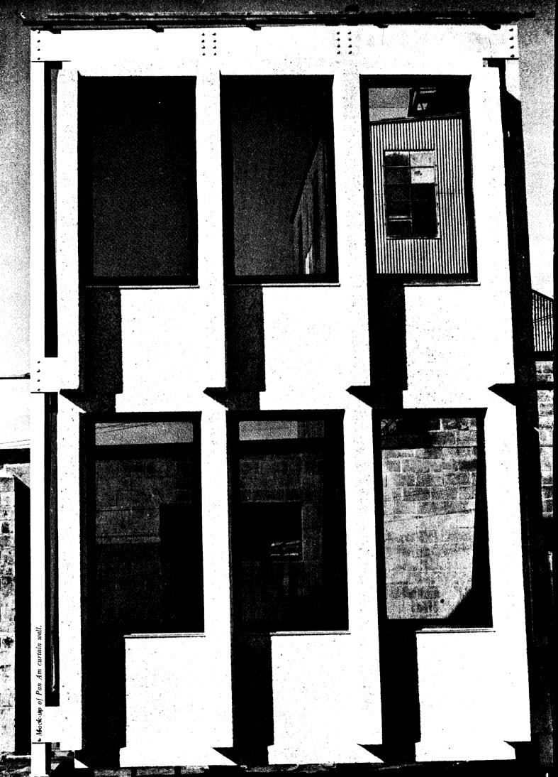
are usually only four corners, there is no call for repetition. Butting two regular panels at the corner is the economical solution. But an engineer cautions that there is greater wind suction at the corners of a building.
