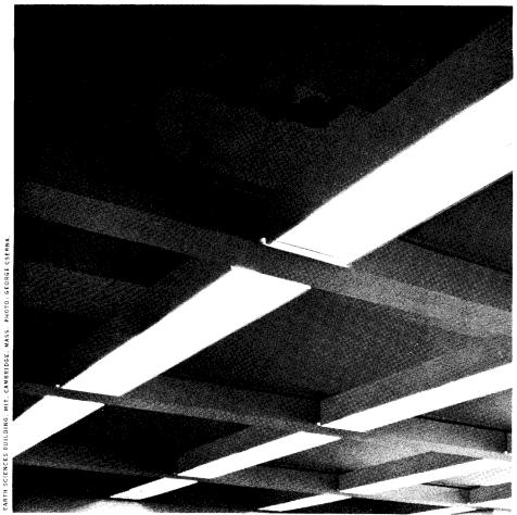
Pierced beams and lighting fixtures create a grid defining the ceiling plane.
