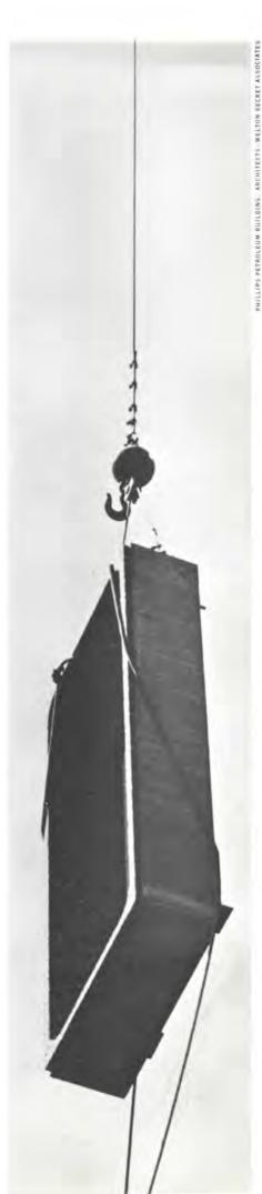
European tower and climbing cranes significantly influenced the spread of precast walls across the U. S. These handling techniques permit contractors to install concrete wall sections without much more difficulty than metal sections.
