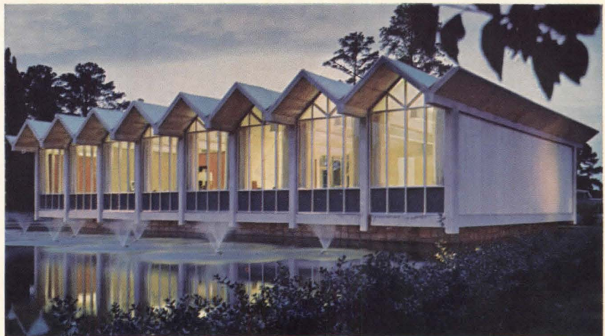
Lutheran Theological Seminary, Columbia, South Carolina. Architect: Lyles, Bissett, Carlisle & Wolff, Columbia.
