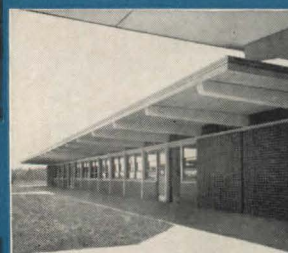
HENRICO HIGH SCHOOL Richmond, Virginia Architect: J. Henley Walker, Jr. AIA
