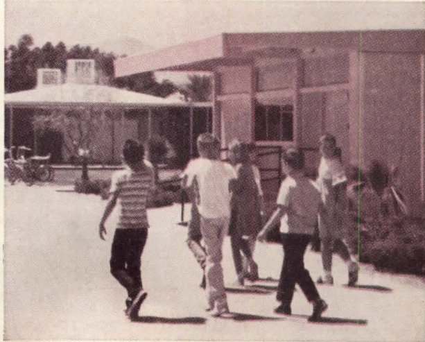
These children will be middle-aged before the 40-year minimum life expectancy of these mobile school buildings expires. A wall core of rigid urethane foam combines structural strength and insulation for long-term economies.
