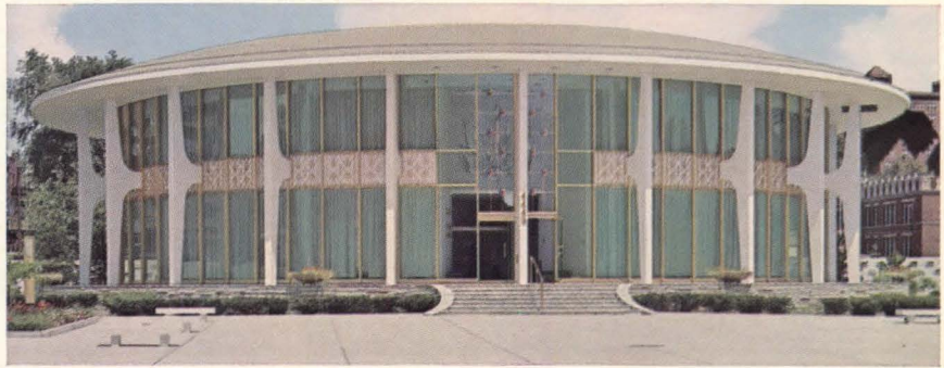
The Chancery Building of the Archdiocese of St. Louis. Architect: Charles Guariglia (Bank Building & Equipment Corporation), St. Louis.
