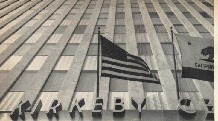
LUSTROUS stainless steel spandrels with No. 4 tinisn alternate with white marble piers at Kirkeby Center, Los Angeles, California. Architects: Claud Beelman and Associates, Los Angeles, Cal. Spandrels, fluted to provide stiffness and eliminate optical distortion, by Construction Metalwork Corp., El Monte, Cal.
