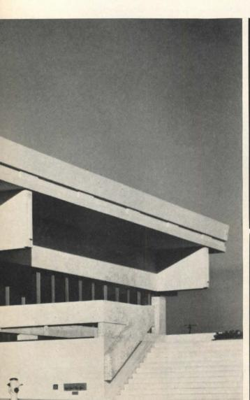
All elements of the Ventura Savings and Loan Association building, except the precast, posttensioned waffle ceiling, were job placed concrete. Interior concrete is natural color and texture. Hand railings are bush-hammered white concrete.
