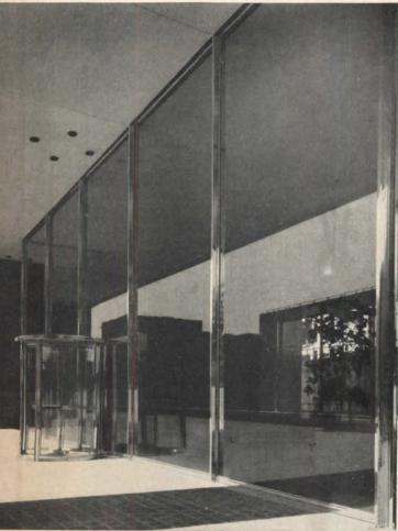
MIRROR FINISHED stainless steel accents red marble and blast-finished granite and provides durability with minimum maintenance in the Sun Life Building, Baltimore, Md. Architect: Peterson and Brickbauer, Baltimore, in association with Emery Roth & Sons. Stainless steel entrances, column covers and window framing: Allied-Superb Bronze Corp., New York, N. Y.
