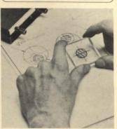
Inked symbols. Stamps mounted on transparent plastic can be inked from special ink pad and applied directly to drafting paper. Ink dries "instantly" on both porous and nonporous surfaces. Any symbol appearing in the American Standards Association catalog, plus other standard designs, are available from stock; custom stamps may also be ordered. Brochure explains use of stamps and shows ex-
