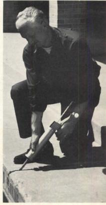
This polyurethane sealant is exceptionally resistant to direct sunlight and the deteriorating effects of water and weather. Standing water will not affect the sealant or its adhesion in the joint.
