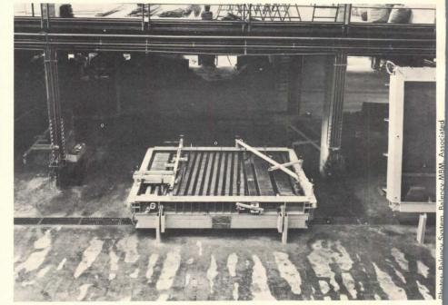
(2, 3) Wall panels are cast horizontally instead of vertically to accommodate inserts and tiled surface.
