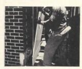
Horizontal supports lock into grooves in edge of 7/8" marble.
