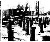
Apiling and form in one, Republic CORWEL® Steel Pile Shell employs helical corrugations to provide amazing stiffness and strength. Welded seam won't part under driving impact. Supplied in needed lengths and diameters. Ask for bulletin.
