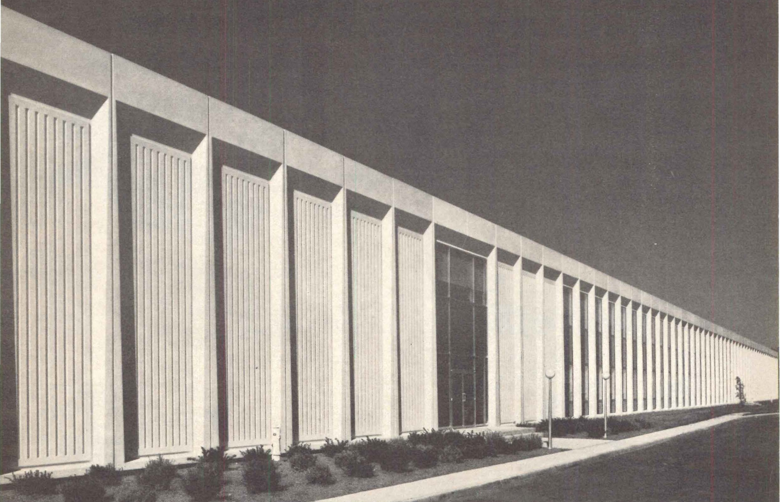
Schokbeton precast concrete curtain wall, Dell Publishing Warehouse, Pinebrook, New Jersey Architect: Frank Grad & Sons, Newark, N.J. Schokbeton by: Eastern Schokcrete Corp.
