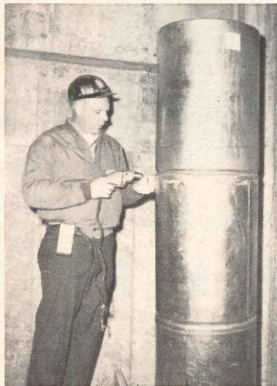
Screw-openings are provided at joints, ingeniously spaced to eliminate adjusting. Three screws secure a section in two minutes.
