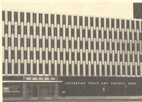
The Jefferson Trust & Savings Bank, Peoria, Illinois Architects: Lankton, Ziegele & Terry Stainless Steel Fabricator: Dawson Metals Products Curtainwall: Rigid-tex pattern 6WL, stainless type 304, by Fenestra
