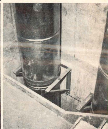
Brackets and drawbands support the stacks at each of first 3 floors and every third floor above. 18" adjustable section below drawband permits expansion, eliminates noise.
