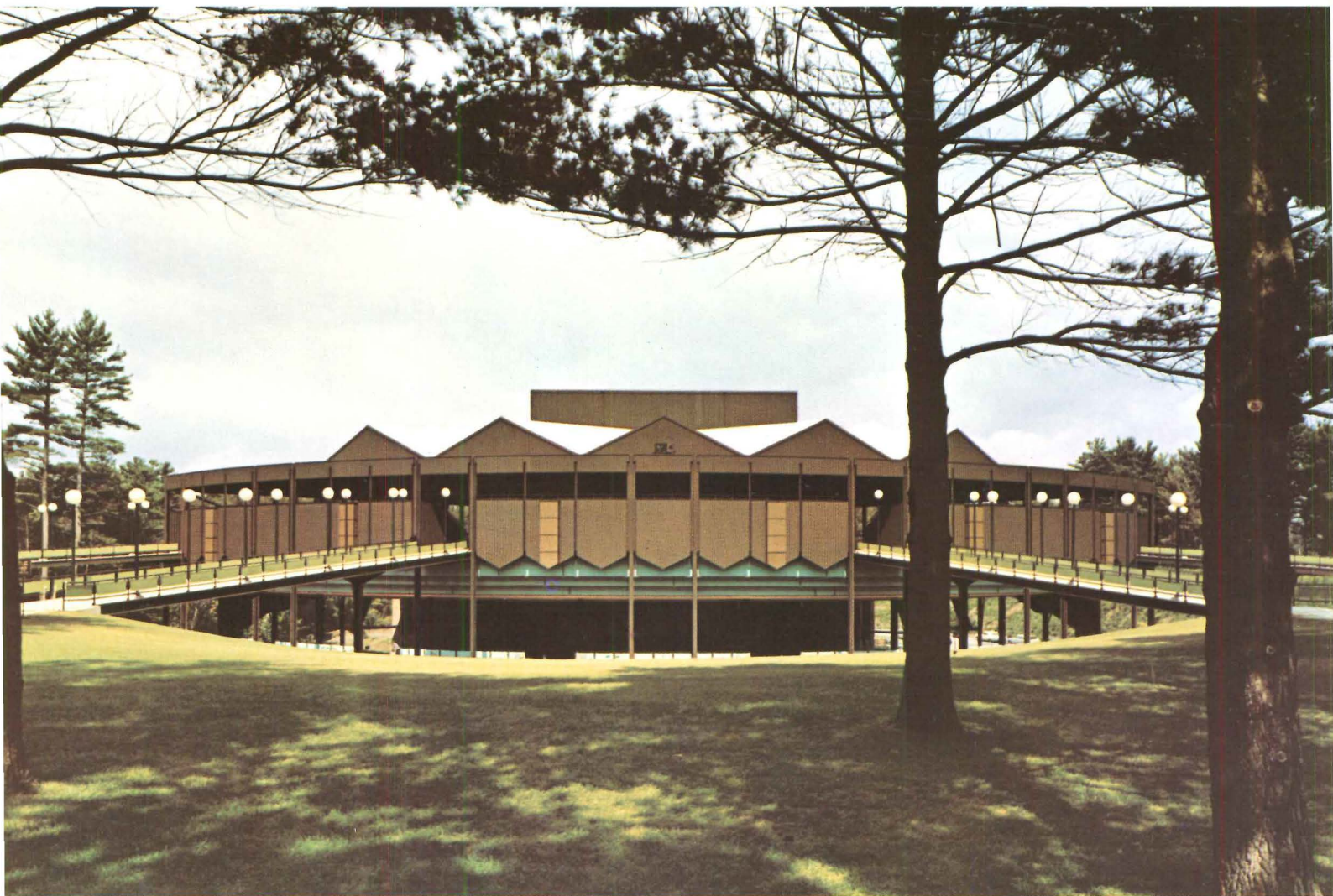
The pleated roof is supported by 126-ft-long trusses, ranging from 16 to 25 ft in depth. Major acoustical element is a steel-framed canopy 100 ft wide and about 50 ft long, cantilevered 50 ft over the audience.
