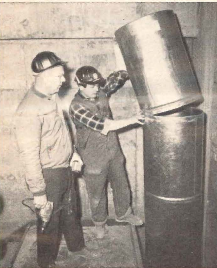
Double steel walls are curled together at upper end of each section, open at bottom. One man easily fits 28 lb. sections together.
