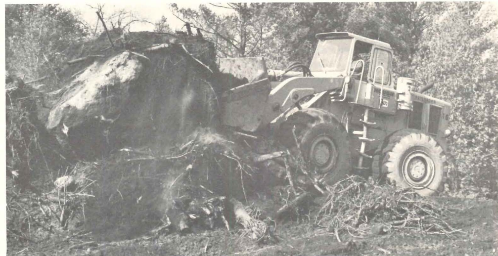
Top: Tractor with bulldozer blade spreads fill. Rear-mounted ripper attachment makes machine double-duty tool. Above: Front-end loader strips and piles soil. Left: Side-mounted backhoe works flush with wall.
