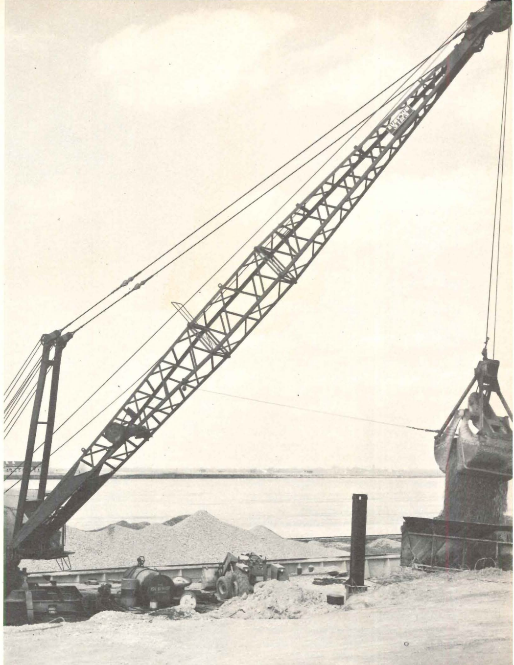
Right: Clamshell loads dump truck. Below: Dragline digs 112 tons with each cast. Lower right: Three cranes with clamshell buckets, a backhoe, and a truck work in close quarters on a crowded city site.
