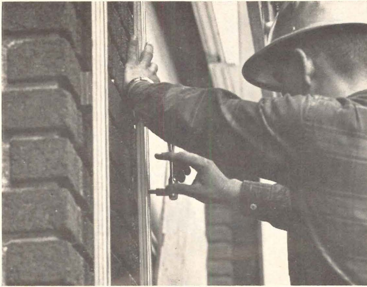
Vertical struts are anchored to existing facade.
