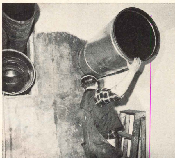
First four pre-assembled sections are inserted from boiler room breeching point thru chase wall. Two men easily handle 110 lb. length.
