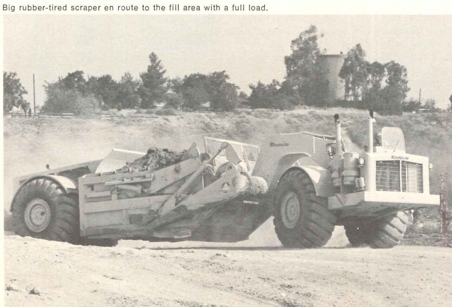
Big rubber-tired scraper en route to the fill area with a full load.
