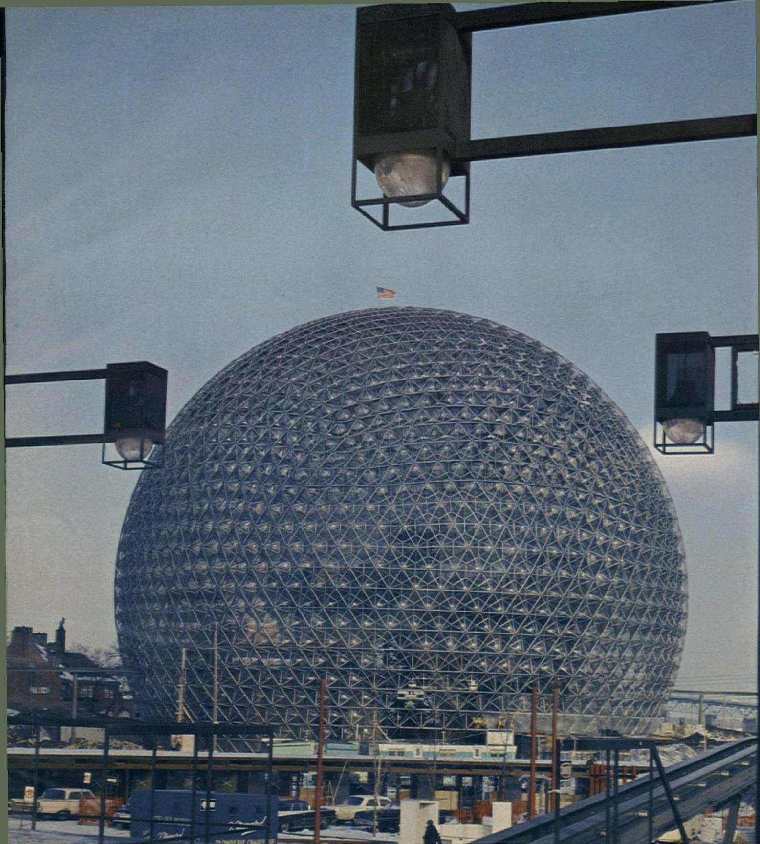
The giant U.S. Pavilion at Canada's Expo '67 is glazed with formed 10' x 12' panels of transparent gray Plexiglas of varying densities. The variation in densities provides graduated control of solar energy and glare. Higher densities are in the upper sections where maximum heat and light control is needed.
