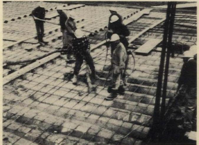
Pumping of concrete to form the slab. Temperature steel and tubes can be seen in place. Tendons are positioned in ribs between the tubes.
