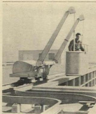
Building maintenance. One-man window-washing scaffold is roof-mounted, and moves vertically, horizontally, and toward or away from the building face. Movement is controlled electrically by the operator. Electrical conductors are encased in steel hoisting cable, thus eliminating separate control cables. Lifting speed is 40 fpm; and horizontal speed is 48 fpm. Patent
