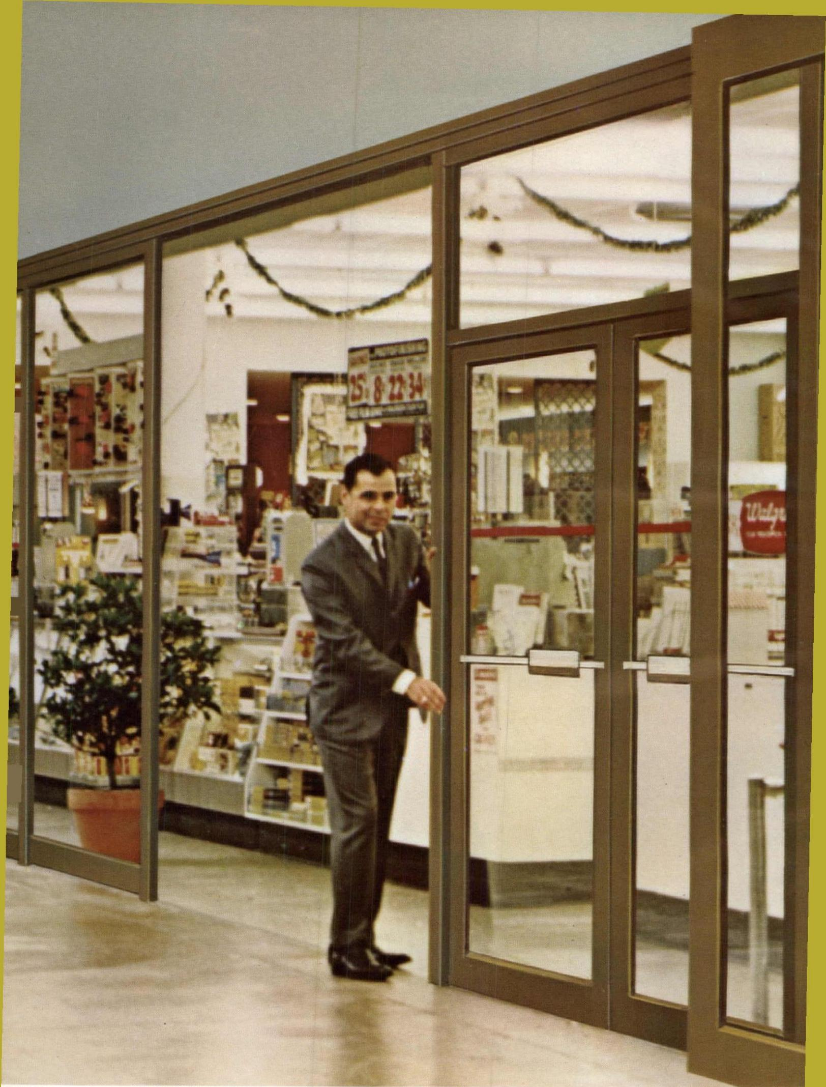
1070 SLIDING FRONT. During inclemency, functions as a normal front with traffic using the swinging doors. In fair weather—or in enclosed malls—the entire front rolls away. Glides on a single flat track set flush with floor. The Kawneer 1040 Sliding Front is similar, but without swinging doors. Panels can turn 90 degrees, permitting flexible storage arrangements.
