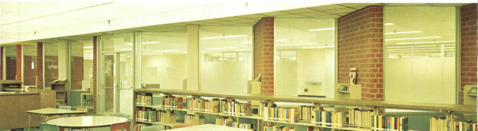
POLISHED MISCO in library windows facing corridor. Mississippi wire glass is used extensively in this structure.
