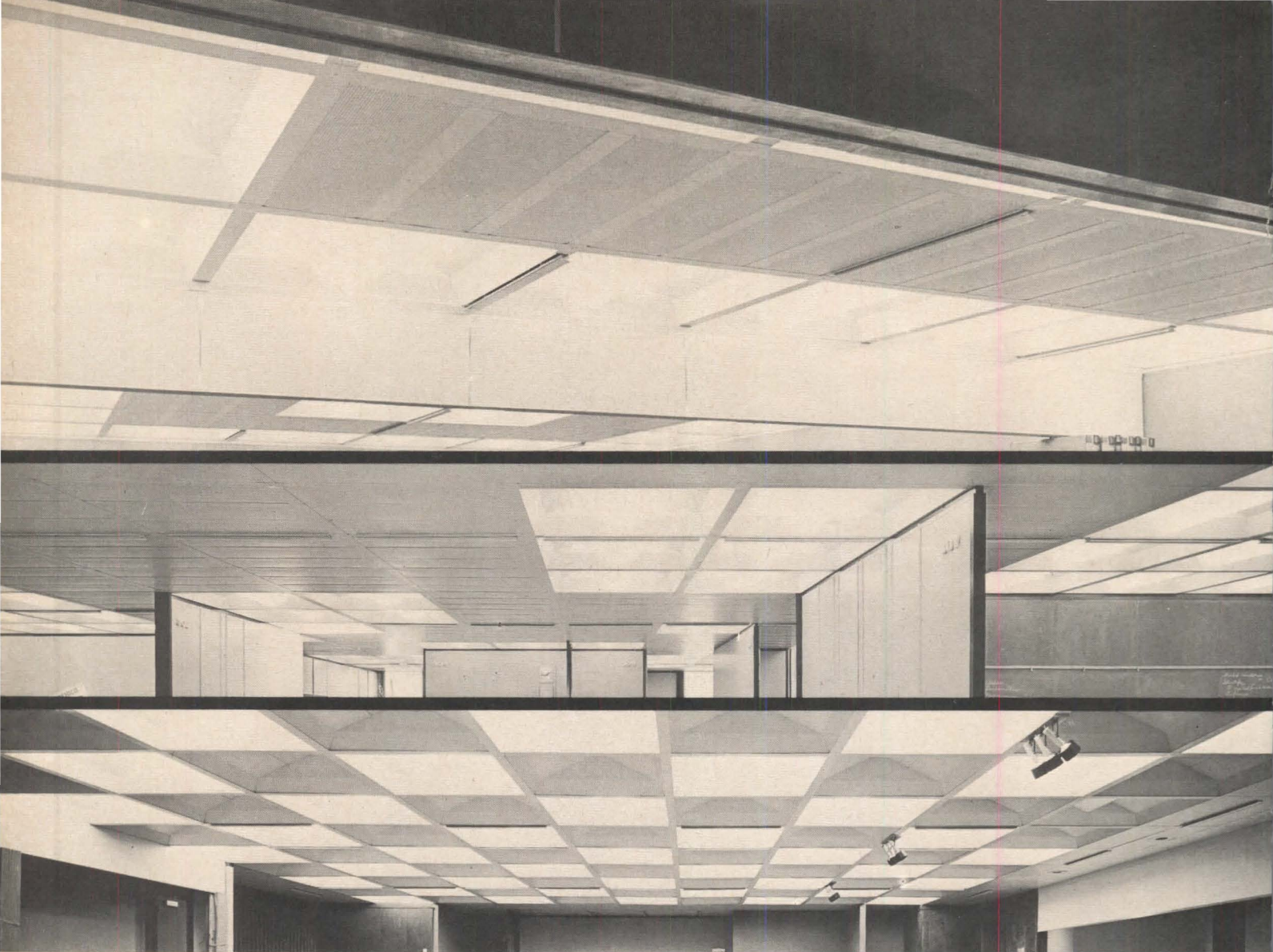
SCSD ceiling and wall systems varied for adjustable school spaces. Ceiling modules are adjusted for multiuse classroom spaces.
