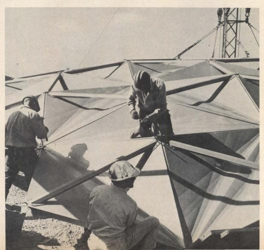
Stressed-skin aluminum panels are formed into a concave "V" shape with 14 creases in a precise pattern that gives the panel its structural strength. Their flanged sides are bolted together at the site, and hexagonal aluminum tubes, or struts, attached to give the stability that allows each panel to act as an individual truss.
