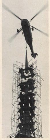
lateral bracing, some provided by concrete platforms that serve as belfries. In all, the tower will hold 56 carillon bells, the largest of which weighs more than 7000 lb. Inside the tower, a winding stairway enclosed in Burma teak will lead to the spire.
