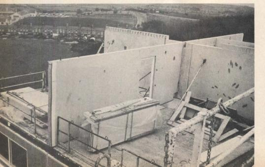
bearing walls is the most practical system for this country. The system is open to maintain separation of trades, but it can be converted to a closed system without significant structural changes by adding industrialized, nonstructural components if and when housing authorities, professions, industry, unions, and the public are ready to accept the concept of factory-made buildings.
