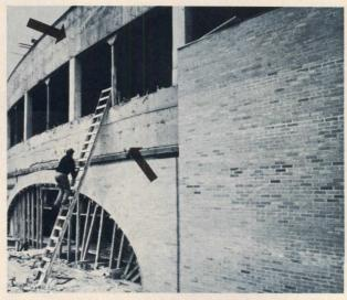
Arrows show location of urethane slab sections which are easily applied to the sub-wall without mastic or fasteners.
