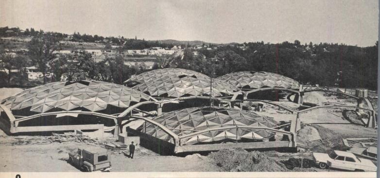
Domes are built on the ground around a grip hoist, then winched into place manually, and fastened to the tension ring. The dome is then completed in place. The steel ring beam is tied across each corner of the hexagon by steel tubes. Attachment of dome to ring beam at corners and at three points on each side of the hexagonal figure is by special struts concealed on the underside of perimeter panels. Open spaces around the perimeter of the domes are closed by half panels or air vents.
