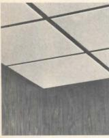
Suspended ceiling with the "homey" look. Two new types of suspended ceiling are for use in residences and offices. In one, wood-grained vinyl is baked on the galvanized steel suspended ceiling components. These are easily installed, since, with system's "Klip-Lock" device, the components can be connected by simply pushing them together. In the other system, tile-like effect is created with a
