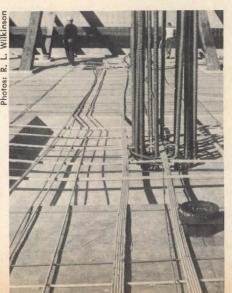
crete beams and slabs, but the others are flat-slab construction. The designers called for 6-in.-deep slabs for the 34-ft spans, and 8-in. slabs for the 41-ft spans. Both systems increase the slab to 10 in. for a 13-ft square around the columns. This enabled ducts and conduits to run within 7 ft of the column centers without passing under the drop panels, where they would lose headroom.
