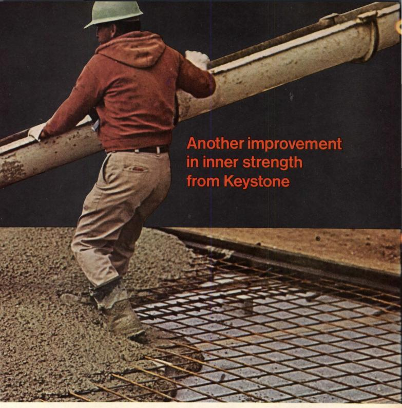
Keyweld sheets and rolls are fast replacing hand-placed, hand-tied rebars to reinforce concrete slabs on grade, floor slabs and walls.
