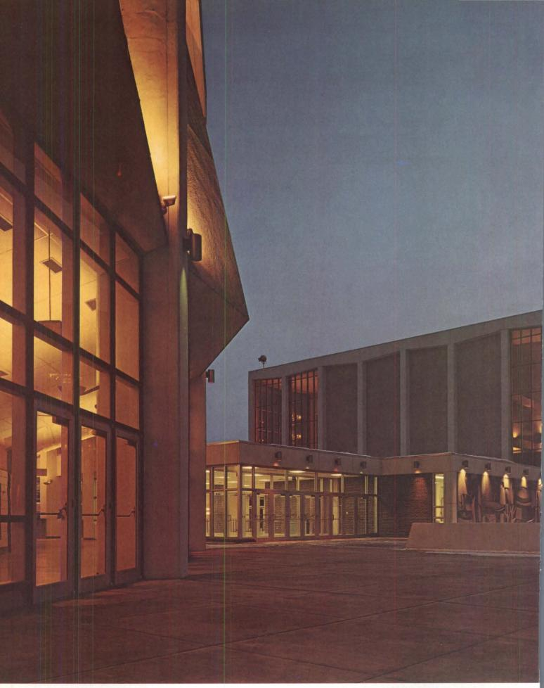
KAWNEER 1600 CURTAIN WALL SYSTEM. Can be specified for both high rise and 1- or 2-story applications with high and wide spans because of extra strength and beefy grid mullions. Available for both plate and insulating glass. Can be
