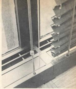
Base of adjustable blind rests inside channel that varies to serve for sliding window-wall onto the court and for fin radiation at exterior walls.
