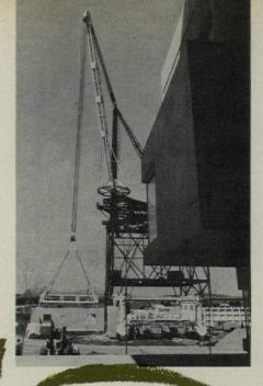
and tied up one crane for handling them. Due to this inadequate arrangement, the house units could not be made weather tight, and this caused damage to the wall and floor insulation, which then had to be replaced. The interior finishing operations were chaotic, and most of the finishing work was done after the boxes were put in place.
