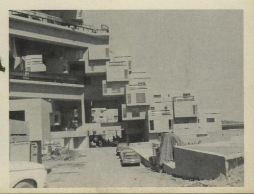
15, 1966, but even with all the drawings for the repetitive geometric pattern of Habitat, the contractor ordered the posttensioning tendons (SS-bars) and other accessories in relatively small quantities.
