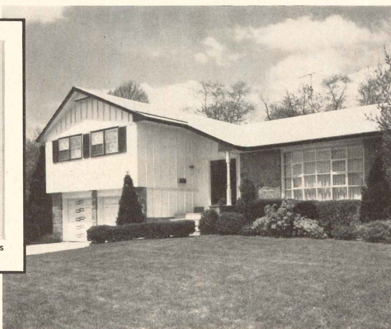
Board-and-batten surfaced with Tedlar provides a handsome, durable, low-maintenance finish.
