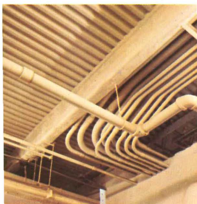
Unusual steel framing system simplifies installation of electrical and mechanical services.
