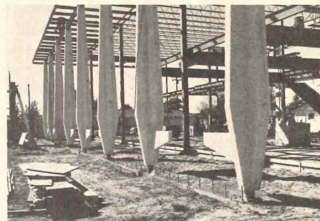
Structural Mo-Sai columns were bolted to concrete foundation and steel roofing system. Wings support Mo-Sai planter boxes.
