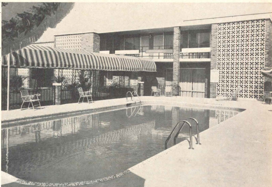
Although two-story motel in Charleston, S.C., appears to be conventional construction, it was built in prefabricated modules transported to the site on highway dollies.
