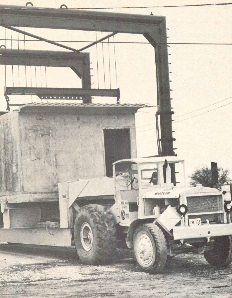
Gantry lifts concrete modules en route to hotel at HemisFair 68. Similar modules cast in same molds are used in two-story housing project in San Antonio (see p. 122).
