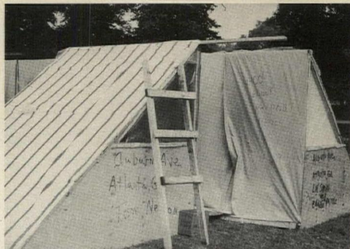
Polyethylene sheets at ridge admit light to A-frame plywood tents, and in hot weather are removed to increase ventilation. Front curtains of paired family units can be draped over extended ridge poles to create protected space between plywood shelters.
