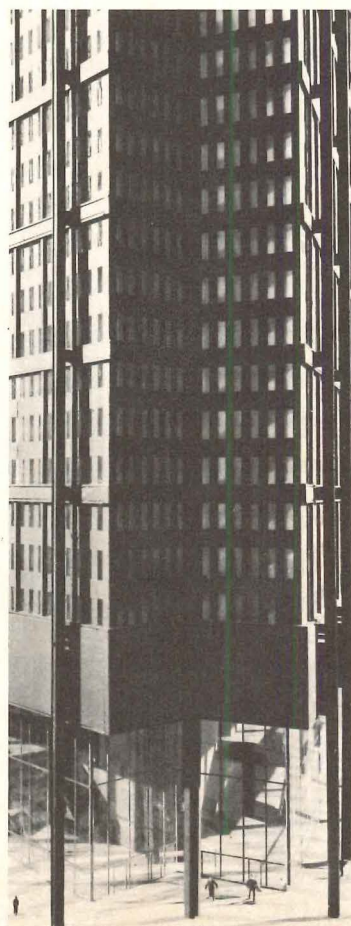
The obvious difficulties of designing a triangular building are apparently overcome in the U.S. Steel Building, Pittsburgh, Pa., by Harrison & Abramovitz. Exterior columns do not obstruct corner views, and notches at apices are deep enough to accommodate private offices.
