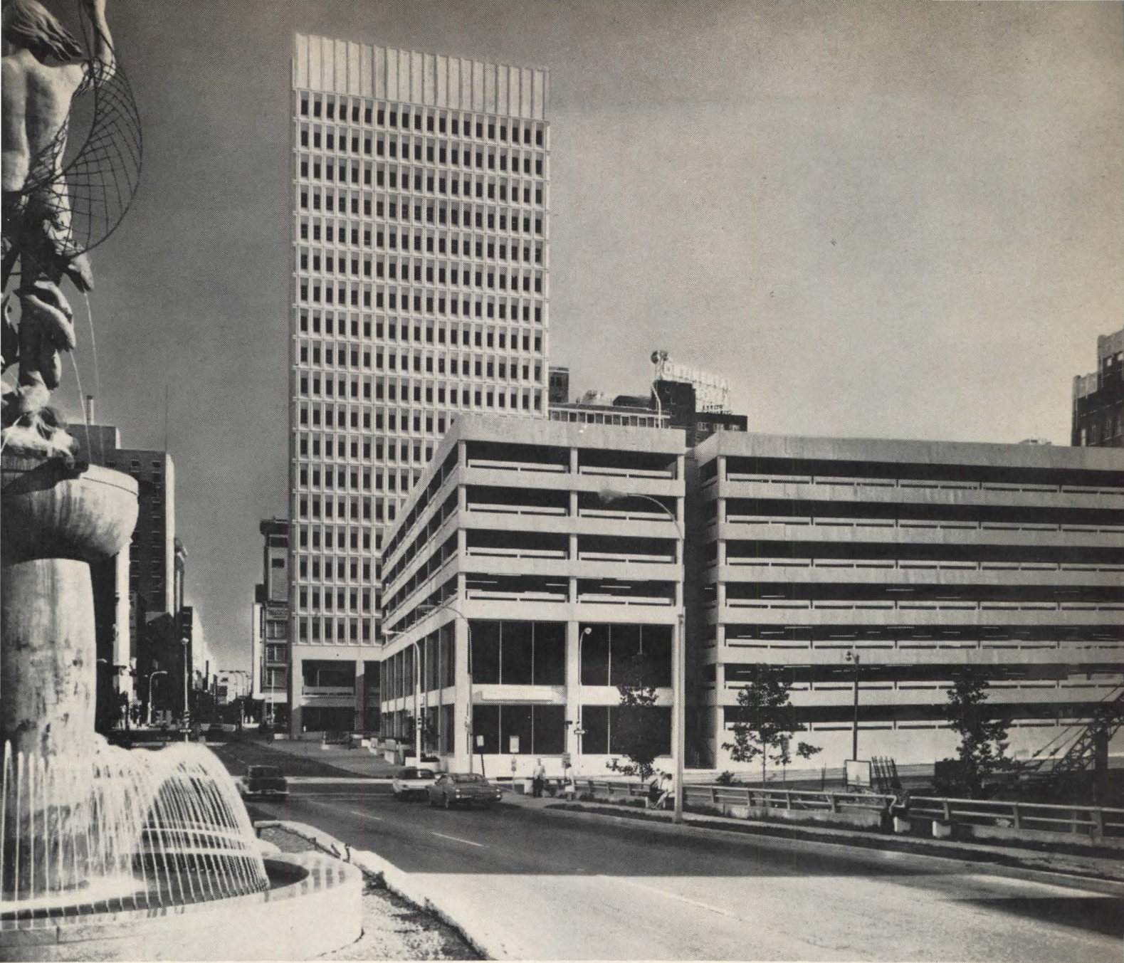
TenMain Center Office Building and Parking Facility, Kansas City, Mo. Monolithic reinforced concrete design/Robert P. Ingram, developer/ Charles Luckman Associates, architects/Marshall & Brown, associate architects/Howard, Needles, Tammen & Bergendoff, engineers/Winn-Senter Construction Company, general contractor/506,354 sq ft of standard Ceco steelform services/ 2,900 tons of fabricated reinforcing bars by Ceco.
