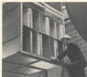
A Koppers sound attenuator in the supply system is examined. Its unique design guarantees noise reduction with minimum air pressure drop.
