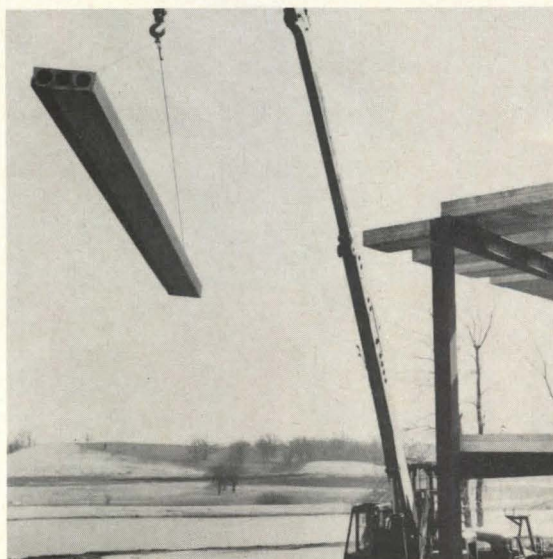
Flexicore erection went ahead during winter months in below freezing temperatures.
